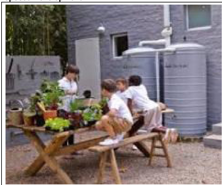
Figure 23: Photograph Showing the Ground Level Rain Water Storage Tanks that can be Used in the Proposed Development.
