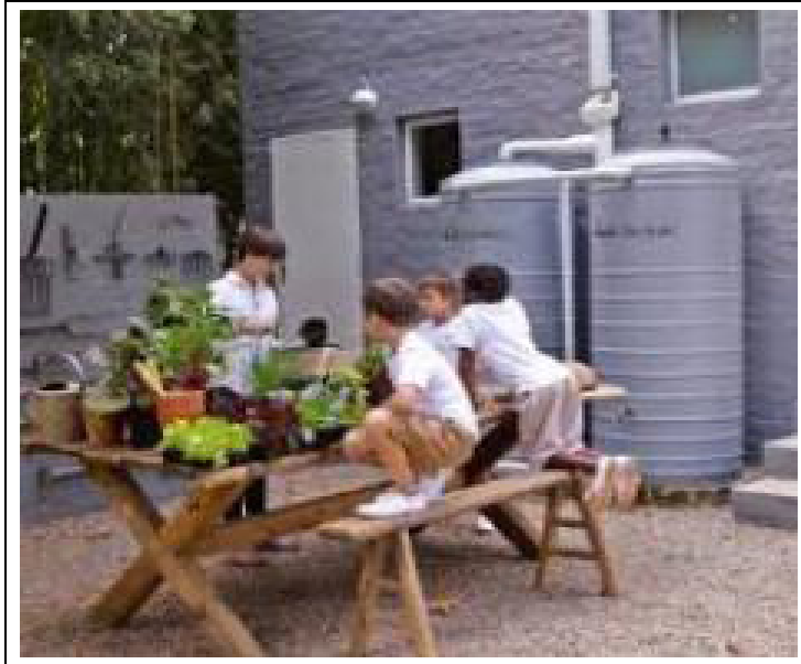
Figure 27: Photograph Showing the Ground Level Rain Water Storage Tanks that can be Used in the Proposed Development.
