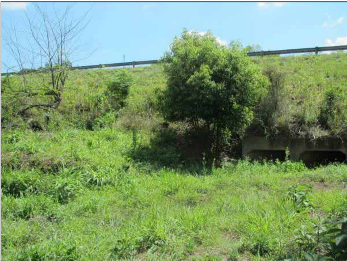
Plate 3. Culvert under N3, silted up and infested with alien invasive species and pioneer indigenous species.
