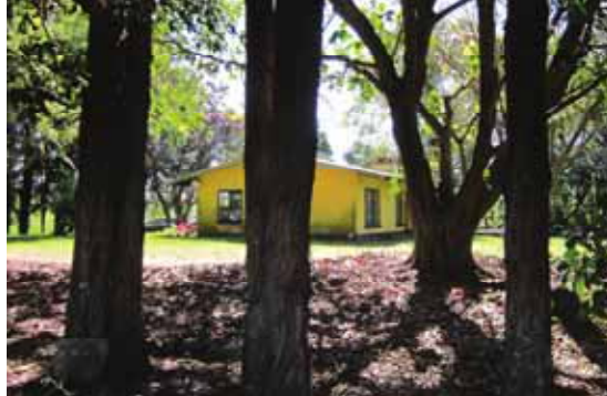
Fig 27: Estate management house 2
