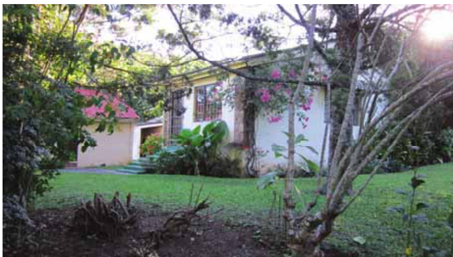
Fig 8: Enclosed portico on double pitched addition to veranda.
