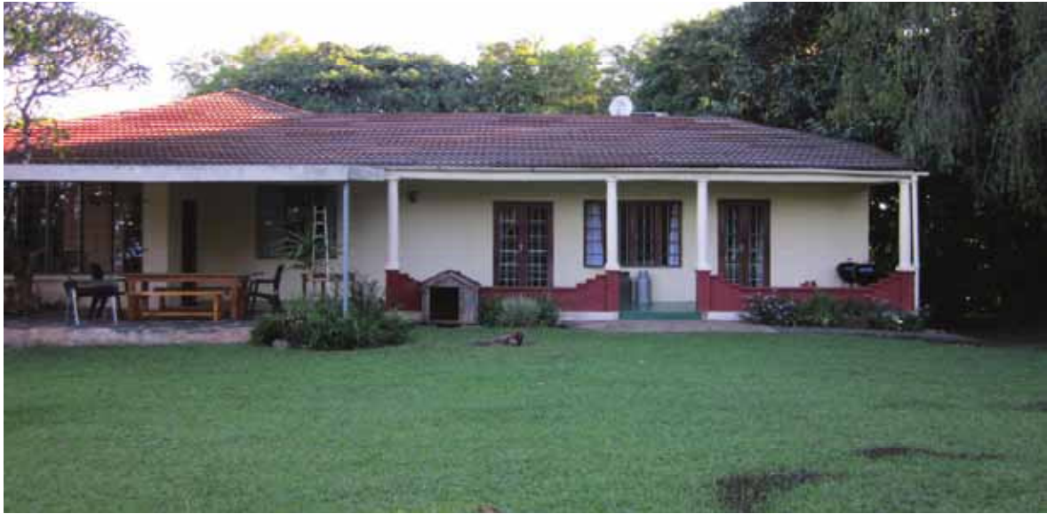
Fig 6: North East Facade of Waterfall Farmhouse
