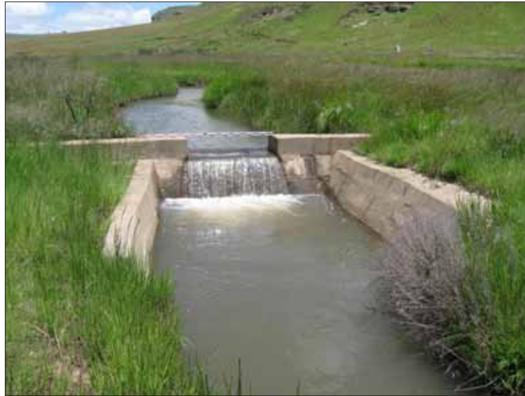
Figure 7-10 Example of a concrete weir
