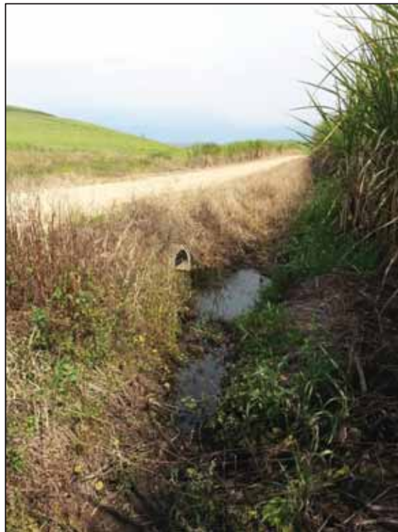
Figure A2-3: Road to be removed from within the wetland and side drain to be deactivated
