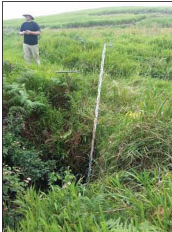
Figure A2- 1: Location of proposed concrete weir at the base of the system
