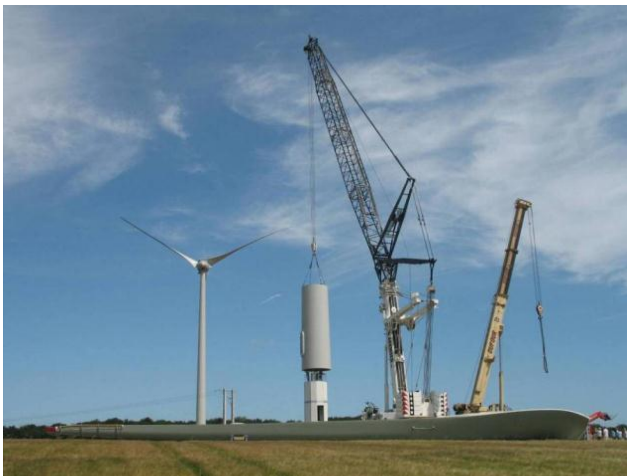
Plate 2-3: Assembly and erection of steel tower sections using cranes.
