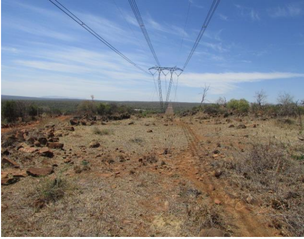
Figure 43: View of power lines across section of the stonewalled site.
