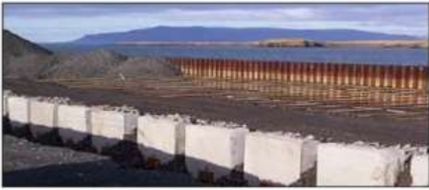
5. Cast deadman and insert tie rods
