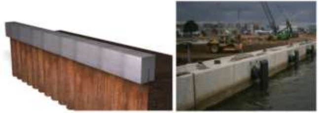
6. Cast capping beam and fender panel
