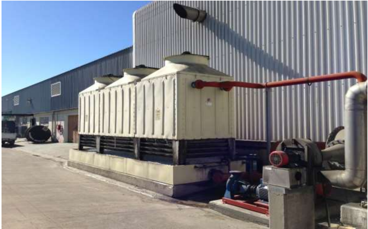
Figure 6: Condensers on the outside of the rendering plant
