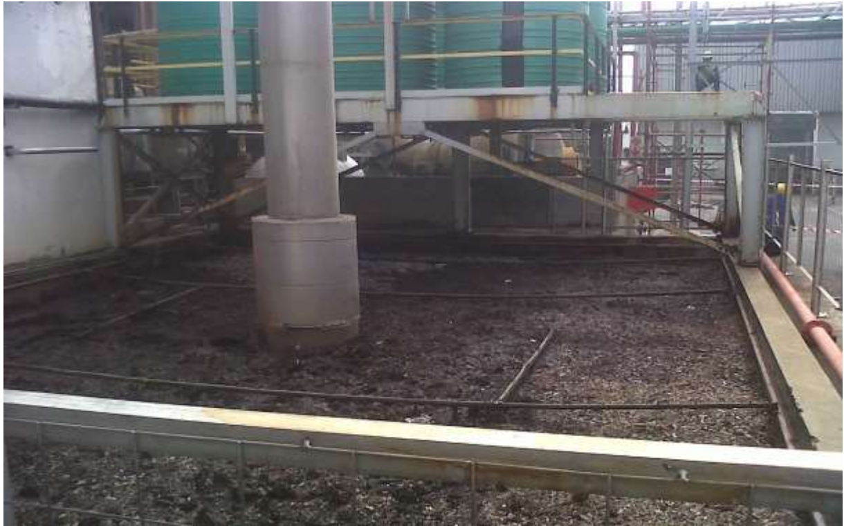
Figure 8: Bio-filter system outside the rendering plant
