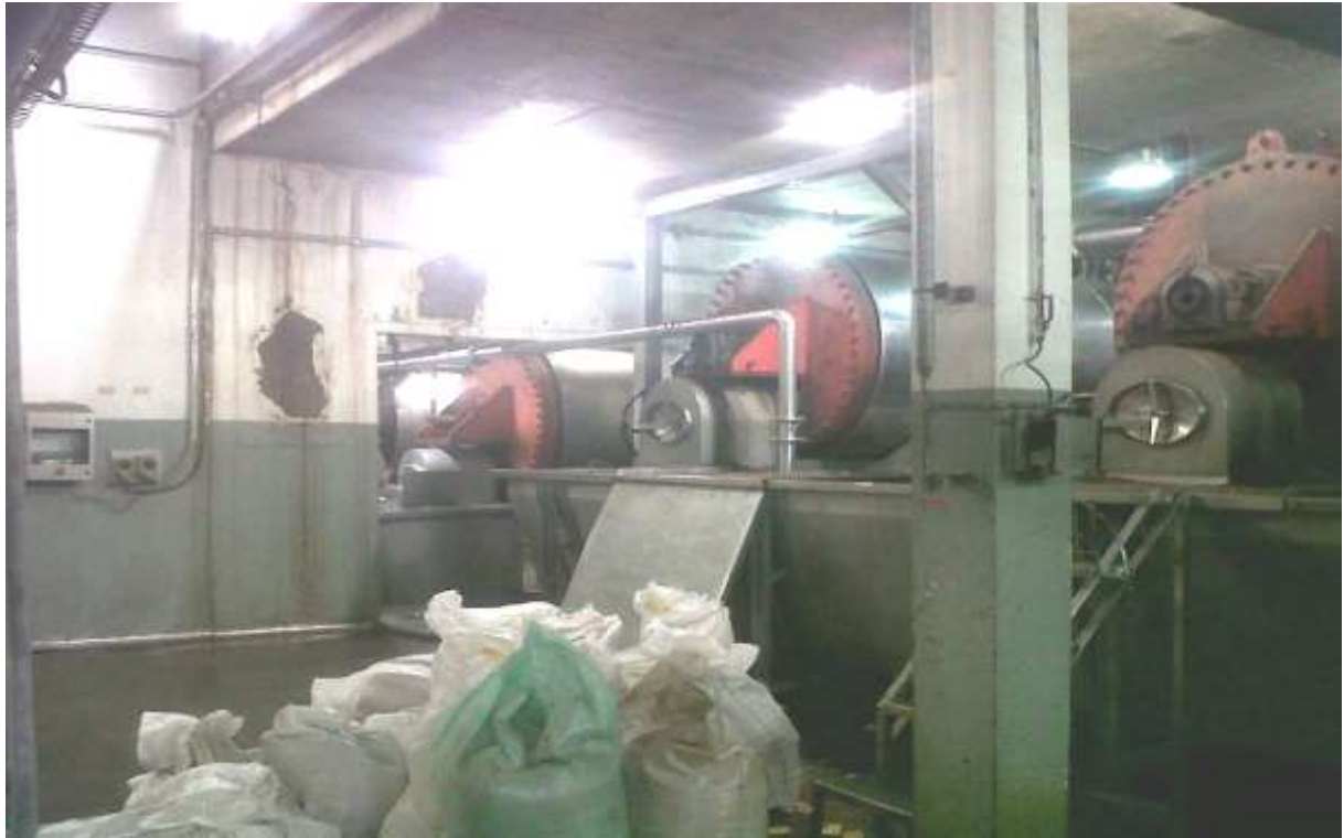
Figure 4: Pressure cooking vessels at the rendering facility
