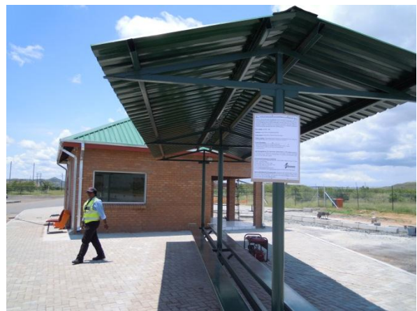
Figure 37: Notice boards placed at the mine entrance
