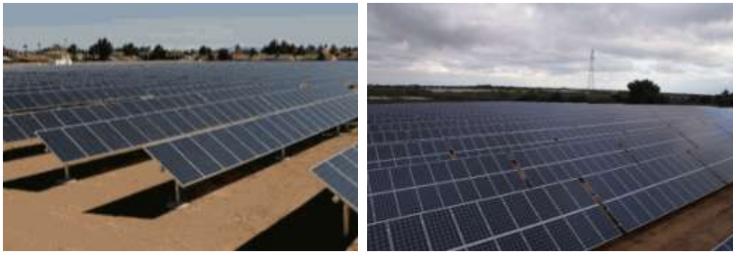
Figure 23: Showing typical positioning of solar arrays in a photovoltaic power generation facility (Solek, 2013).
