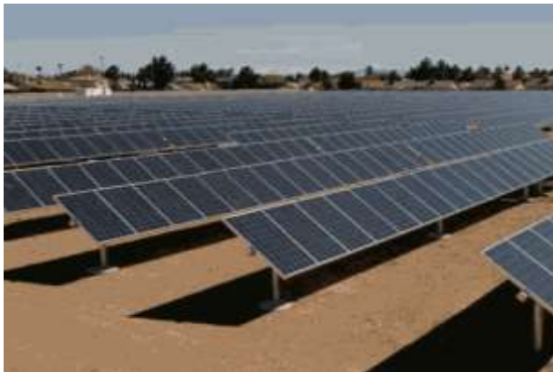
Figure 21: An example of a single axis tracking system. NB – The final tracking technology will be only be decided at a later stage during the detailed design.
