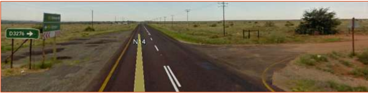
Figure 38: Showing access to the D3276 from the N14.
