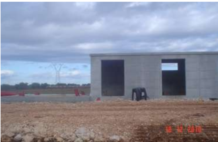
Figure 28: Typical example of auxiliary buildings under construction (Solek, 2013).
