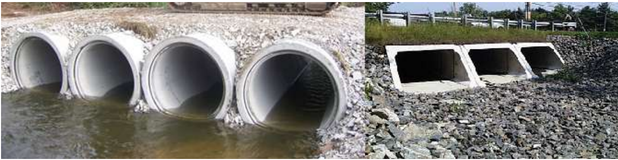
Figure 29: Showing examples of temporary measures for the potential crossing of the main drainage channel on site (Solek, 2013).
