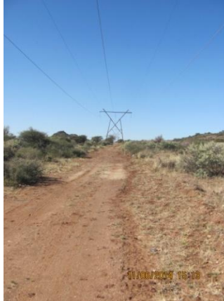
Figure 13: 132kV wooden-lattice power line from west, forming the southern boundary of the proposed solar site. A section of this service road (along the southern boundary) forms part of the Option 2 access road from the south.
