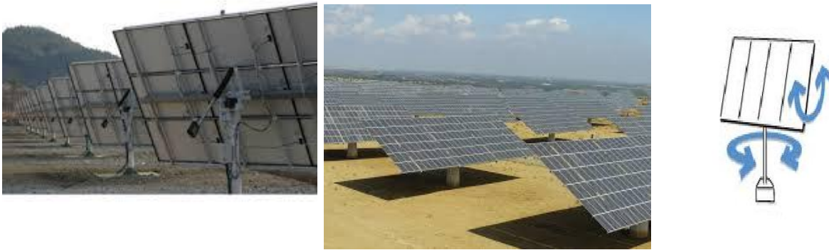
Figure 5: Examples of double axis PV tracking systems.
