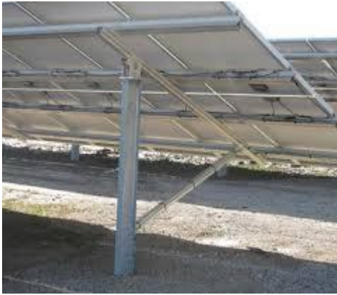
Figure 7: Typical rammmed or screwed method of installation.
