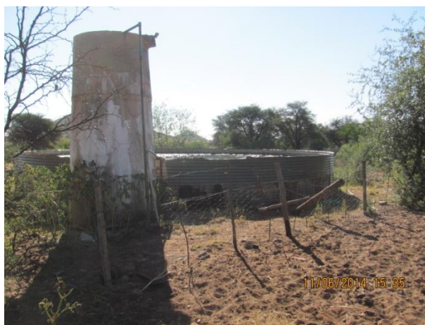
Figure 19: One of two water reservoirs connected to borehole / solar pump.
