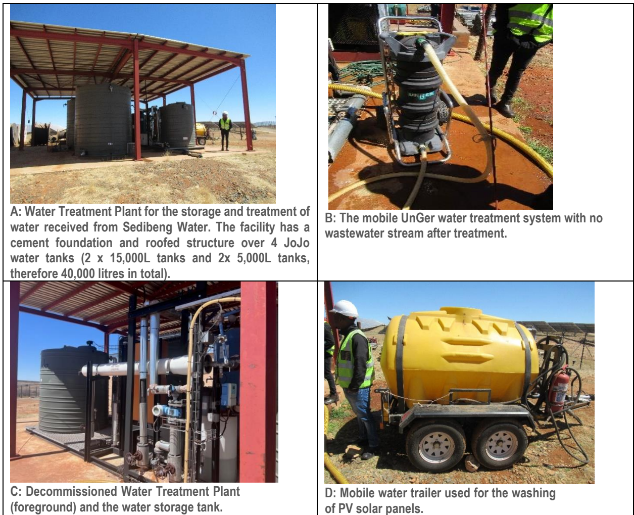
Figure 19: Water Treatment Plant
