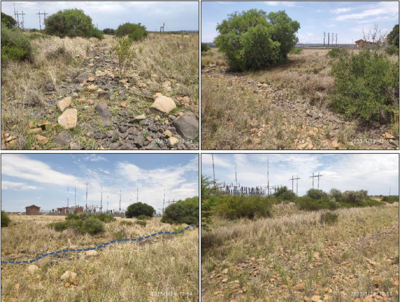
Figure 37: Rocky streambank of the non-perennial stream (top) and a view of the substation from west of the non-perennial stream (bottom) (Vegetation Review, 2023)
