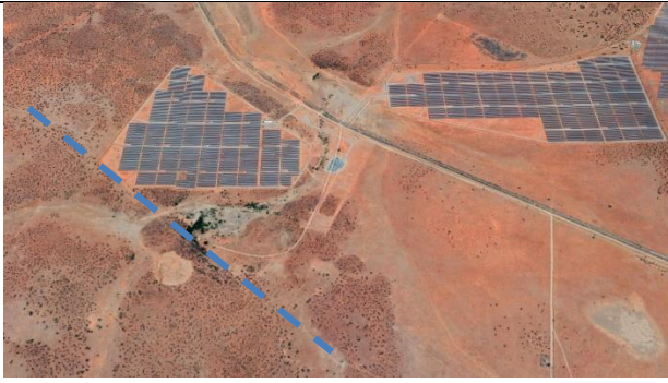
A: Location of Lesedi Solar Power Facility (south solar field on the left, and north solar field on the right), in 3D relief, showing Eskom transmission line (blue dash line) (Source: Google Maps, 2021).
