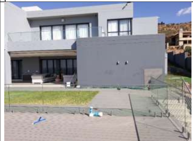
Photo 5: South west looking towards the main house.
