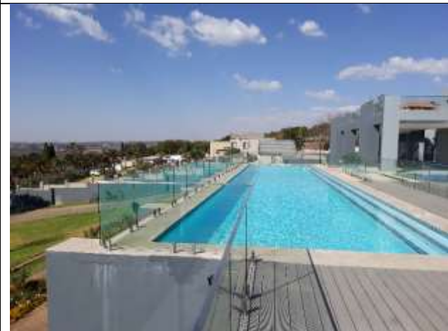
Photo 3: South east looking over the swimming pool.
