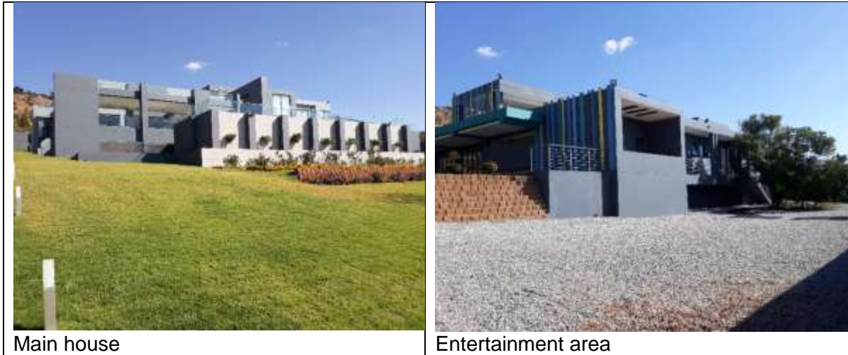
Figure 3.1: Two main structures on the property
