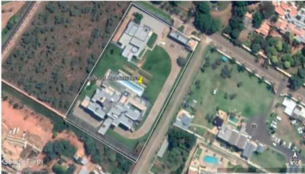
Figure 3: The developed site and the neighbouring stand to the west, covered with natural Protea caffra -dominated veld.
