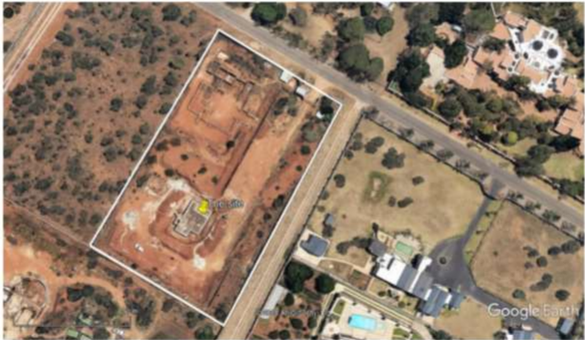
Figure 3: Detailed view of the site during construction.
