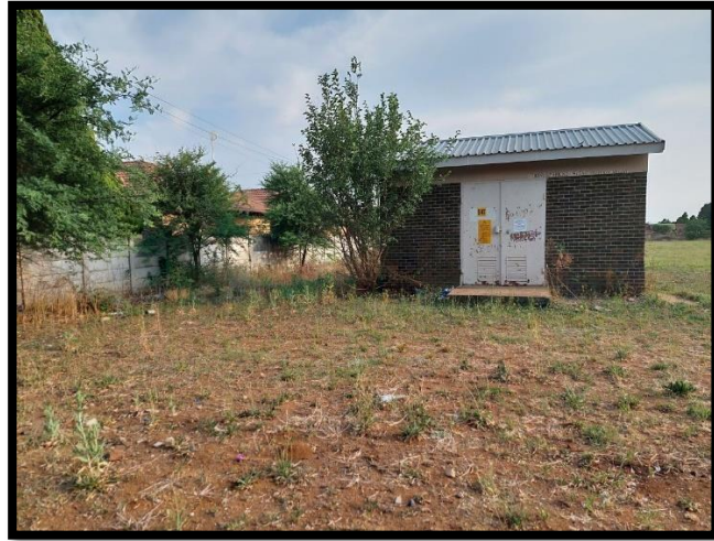
Photograph 3: There is an electrical substation on site
