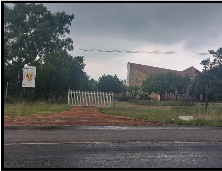
View of adjacent church complex
