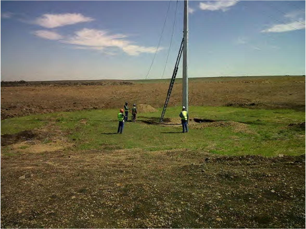
Base of the mono-pylon/Tower
