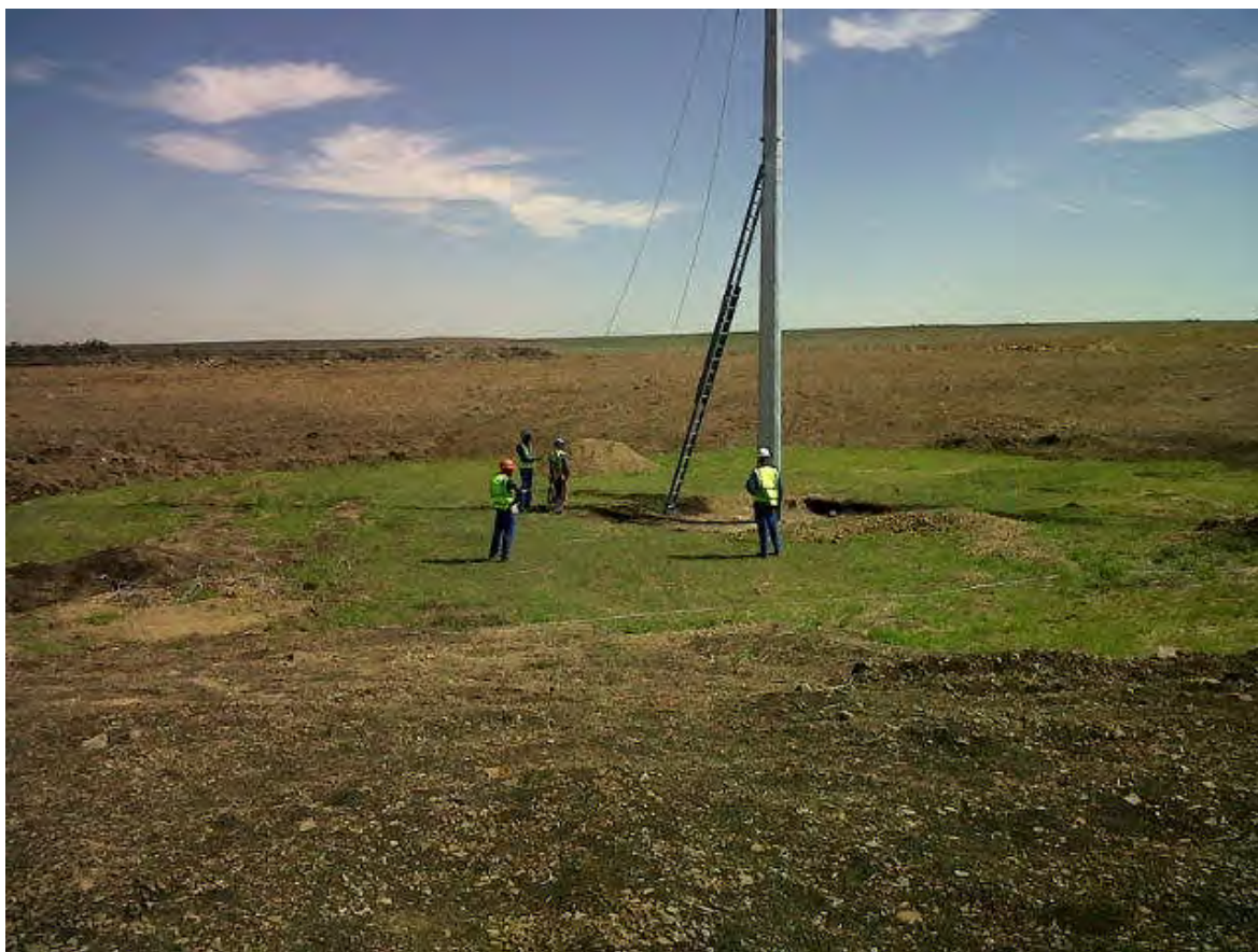
Base of the mono-pylon/Tower
