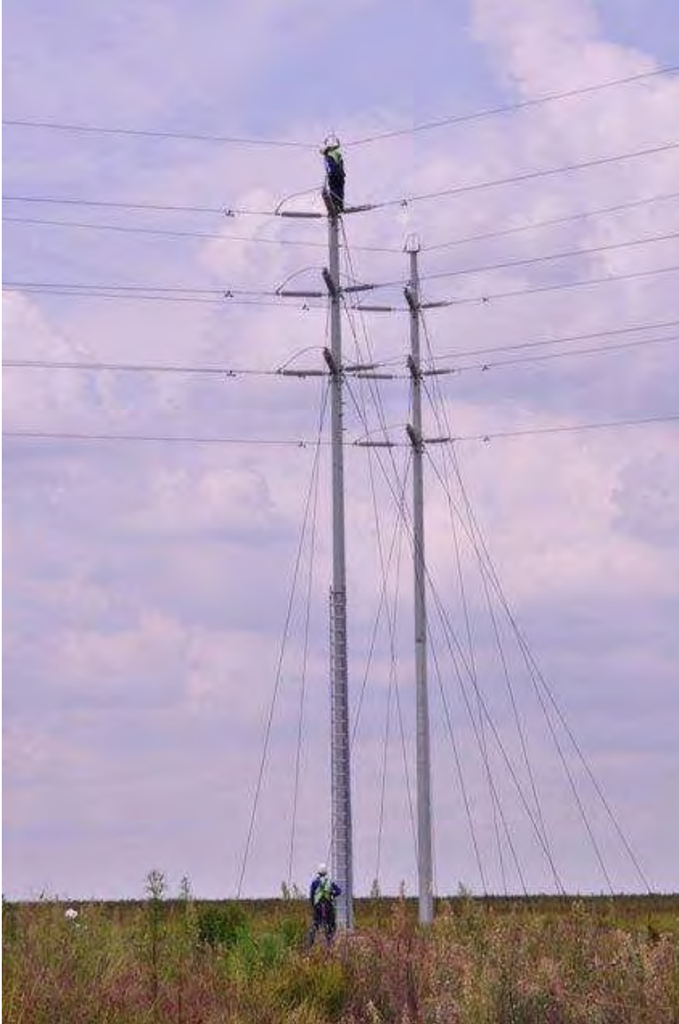
Example of mono-pylon/tower to be used
