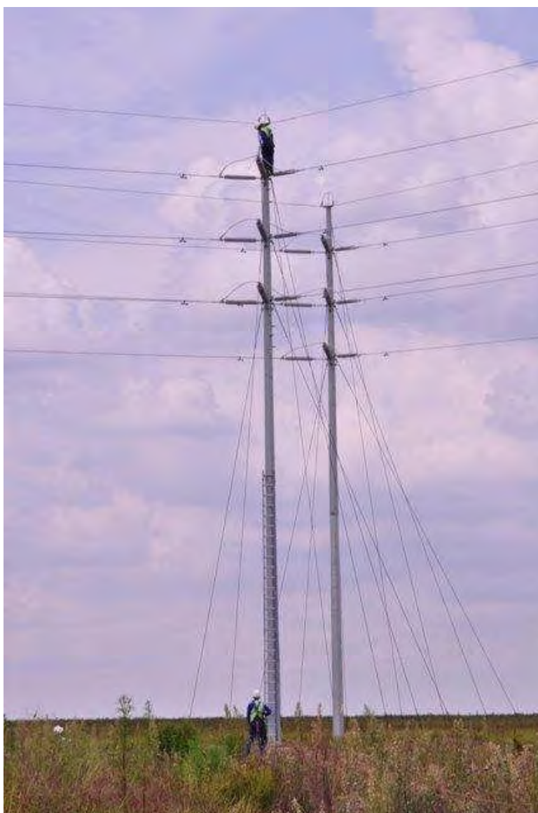
Example of mono-pylon/tower to be usdd
