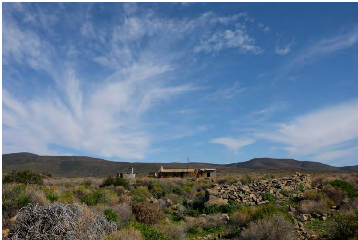
Figure B.35: Historic stone (foreground) and brick (background) buildings with recent alterations and additions serving as labourers' residence at Boplaas on upper reaches of Uriasgatrivier Valley CLA (photo courtesy of Hearth Heritage)
