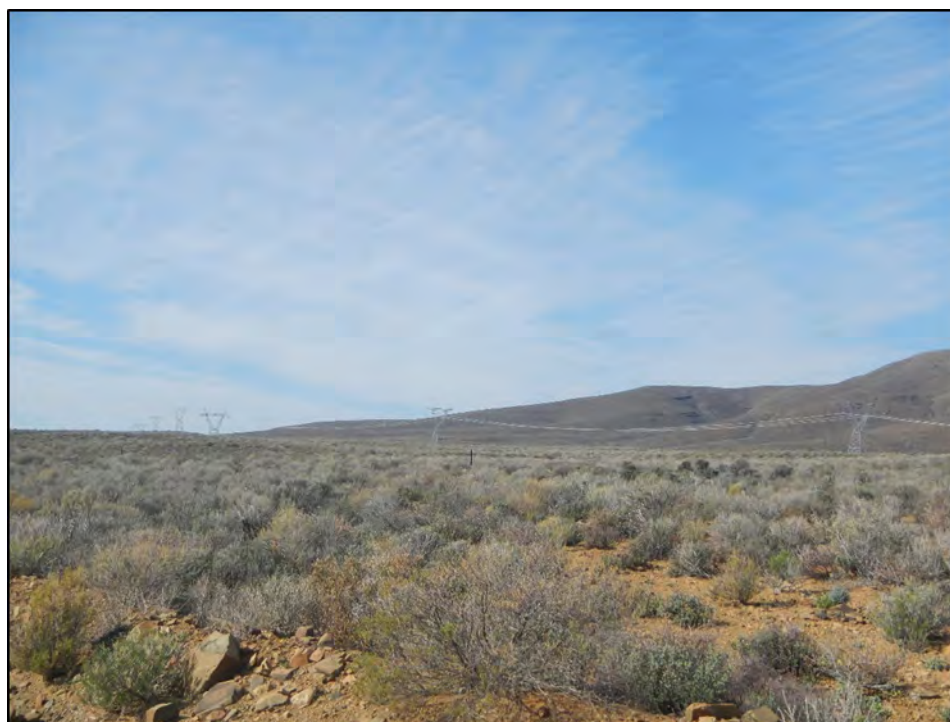
Figure D.5: Typical view of some of the existing high voltage power lines which traverse the southern section of the study area (photo courtesy of SIVEST)
