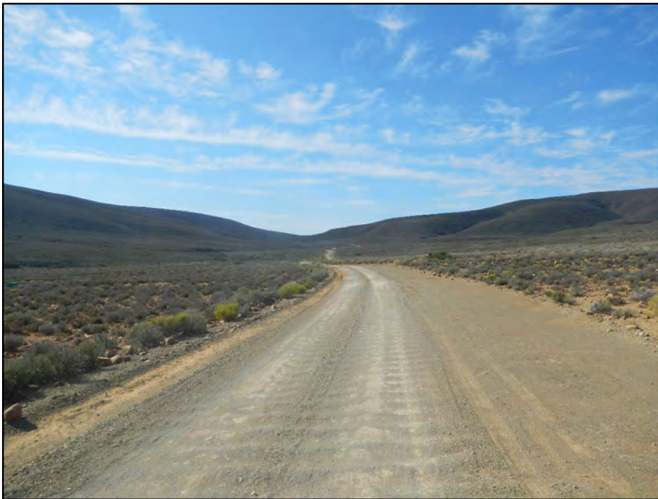
Figure D.6: Typical view of the R356 Regional Route (photo courtesy of SIVEST)
