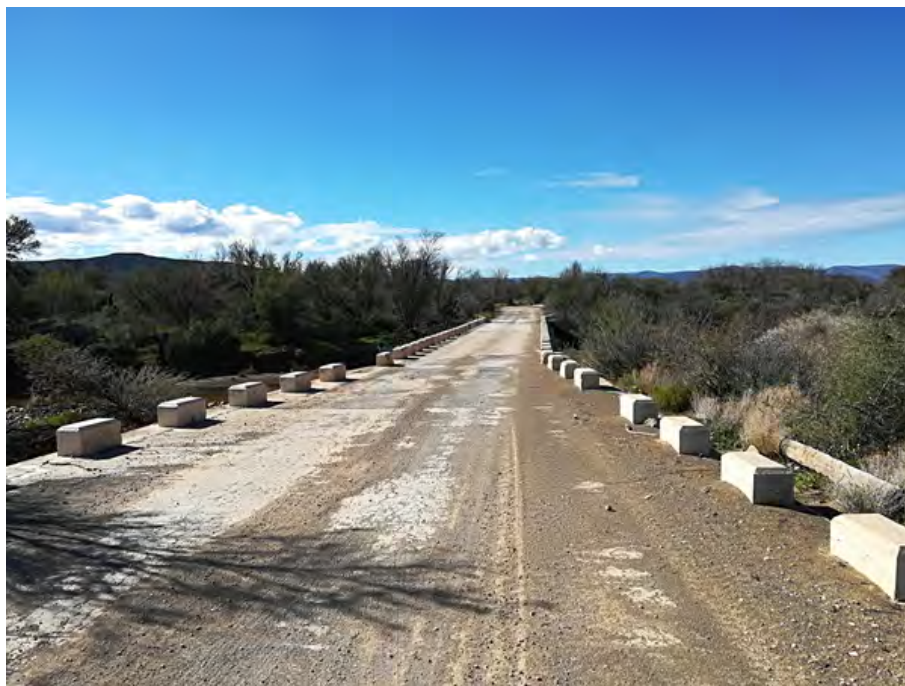
Figure D.35: Narrow bridge on DR02249
