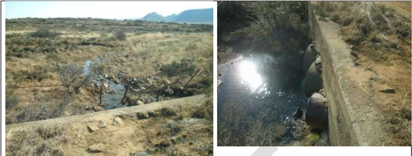
Figure 2.8. Access road bridge over the Wolwekop Stream
