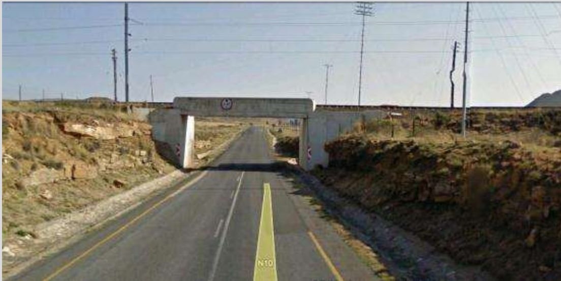
Photo of the Flonkers rail over road bridge that will be upgraded.
