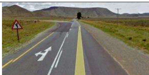
Photo 10: The endpoint of the proposed road upgrade.
