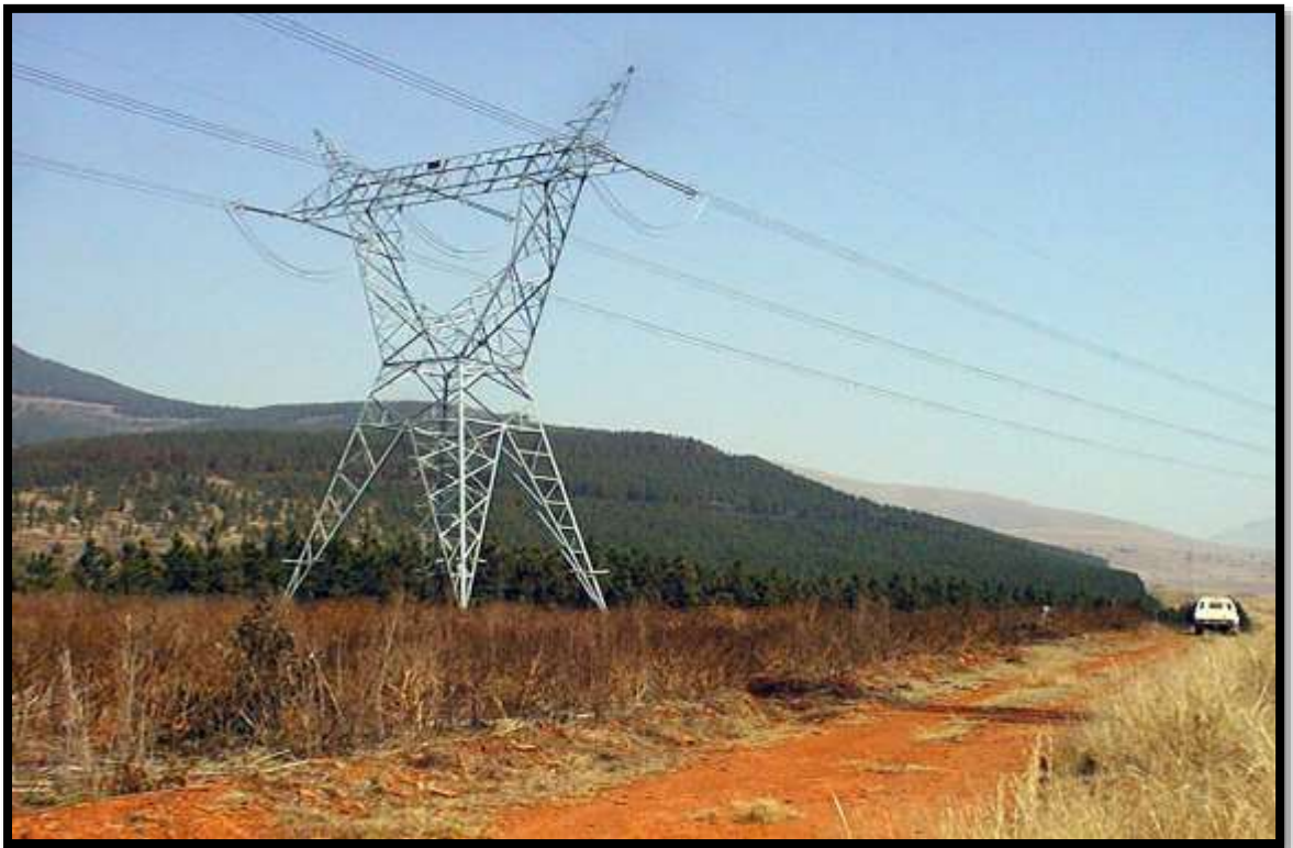
Figure 9: Bend/Strain structure
