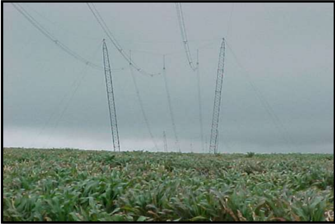
Figure 10: Cross Rope Structure
