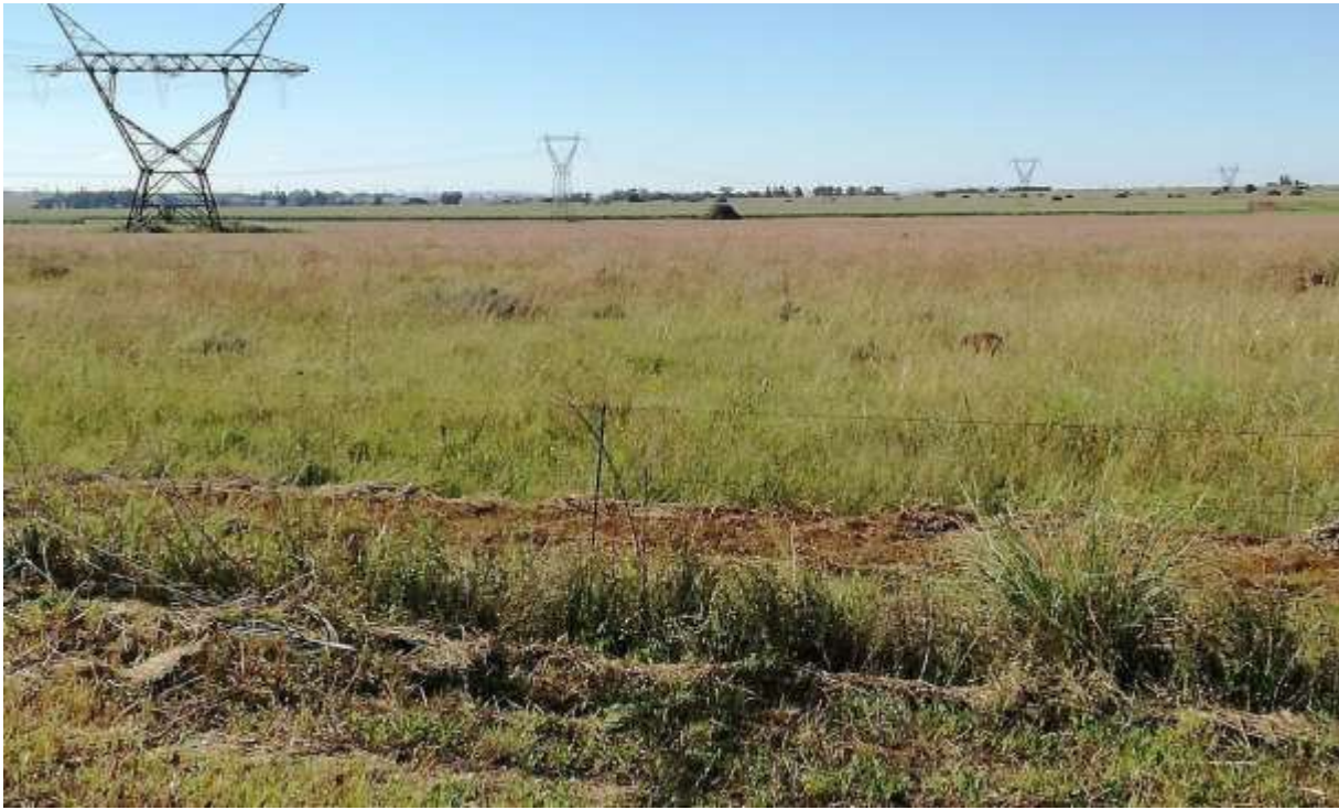
Figure 108: View of existing Powerline from Pluto substation to Watershed substation
