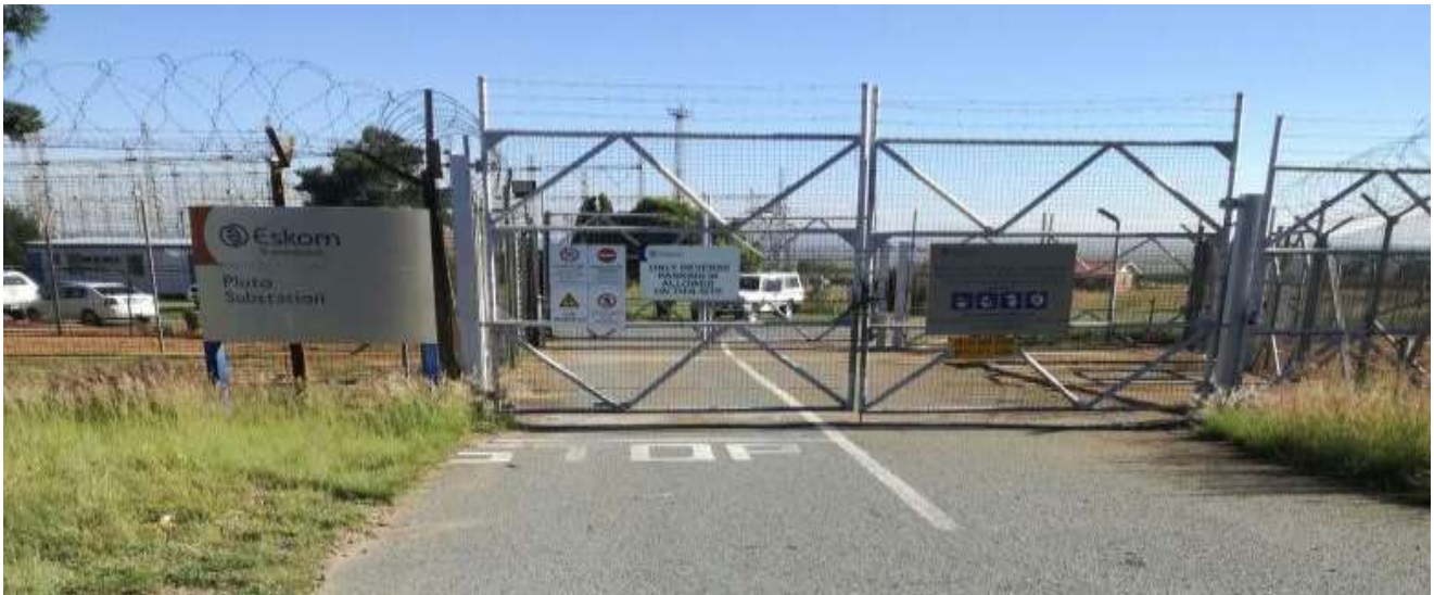
Figure 102: Pluto Substation in Gauteng
