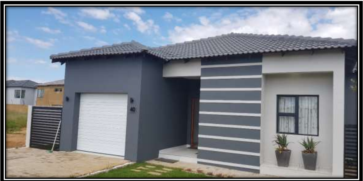
Photograph 2: Phase two (2) involve the construction of single story residential houses
