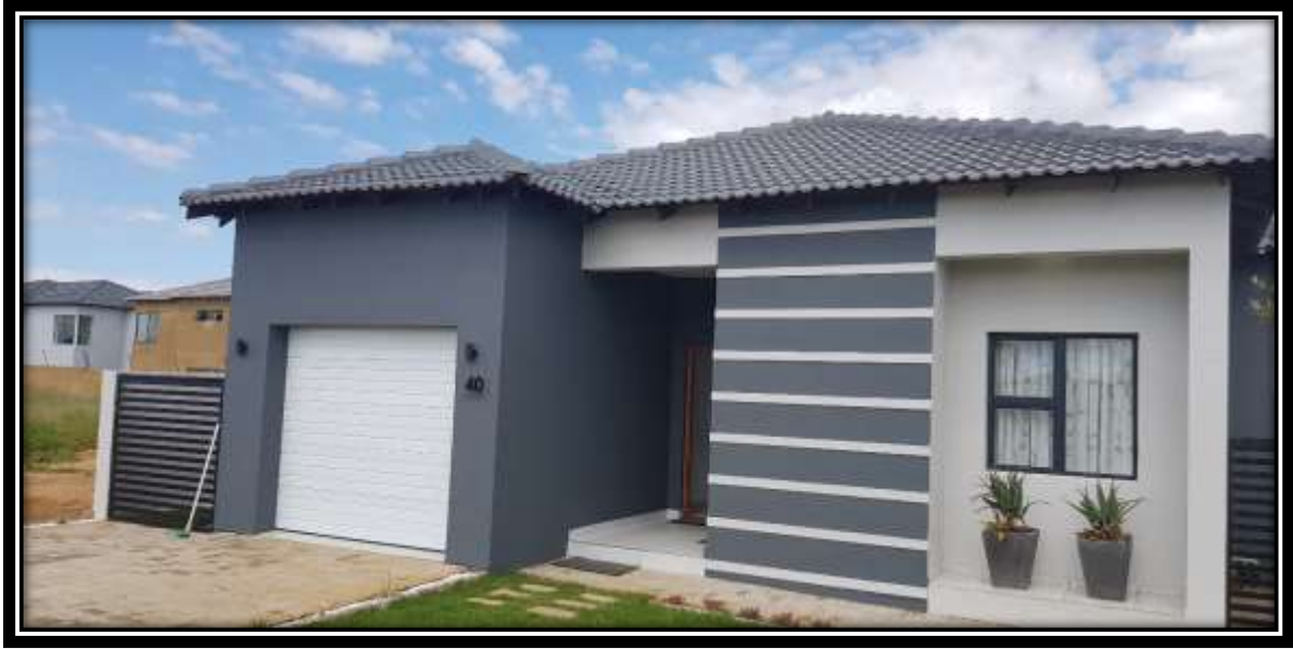
Photograph 5: Phase two (2) involve the construction of single story residential houses
