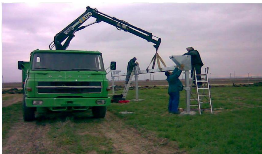
Figure 2.6 Mounting of the frame for the PV panels (Courtesy of Igeam, 2011)
