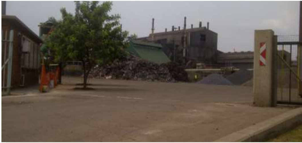
Figure 4: Illustration of steel shaving stockpiles (1)
