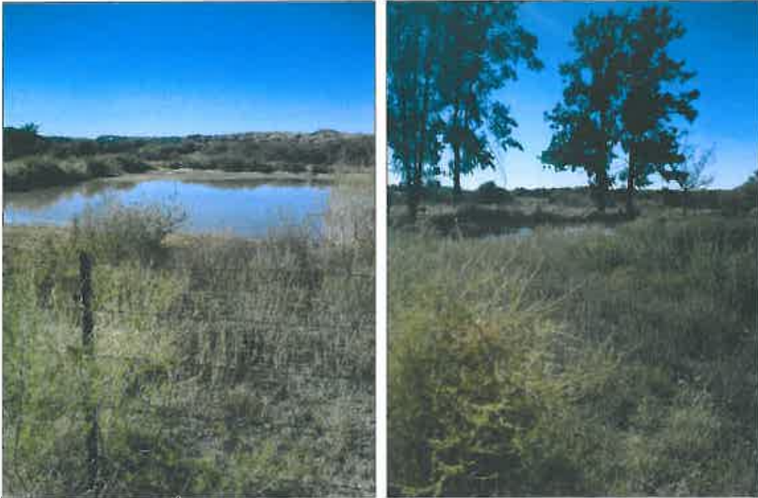
Photos 10 and 11: Old sewage dams present on site that will need to be rehabilitated.
