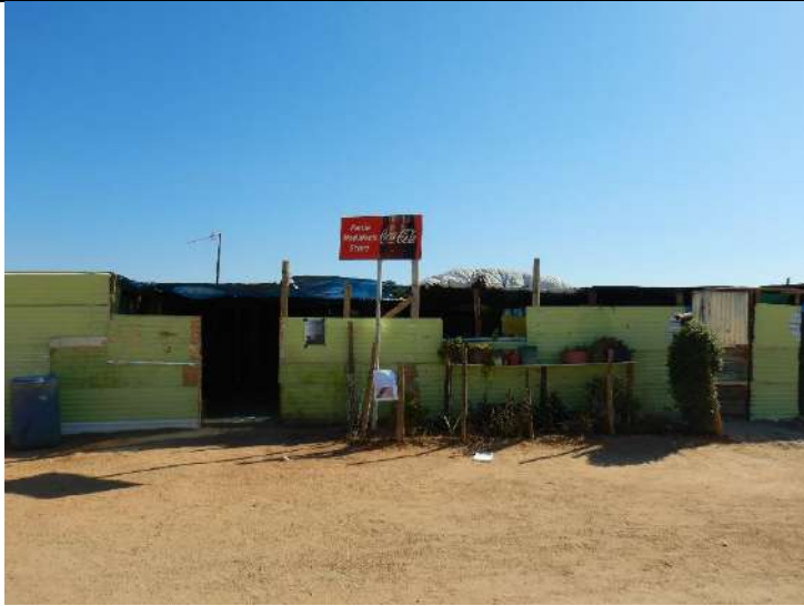
Figure 17: A3 Poster placed against the fence at Fanie Madidach Store on site.
