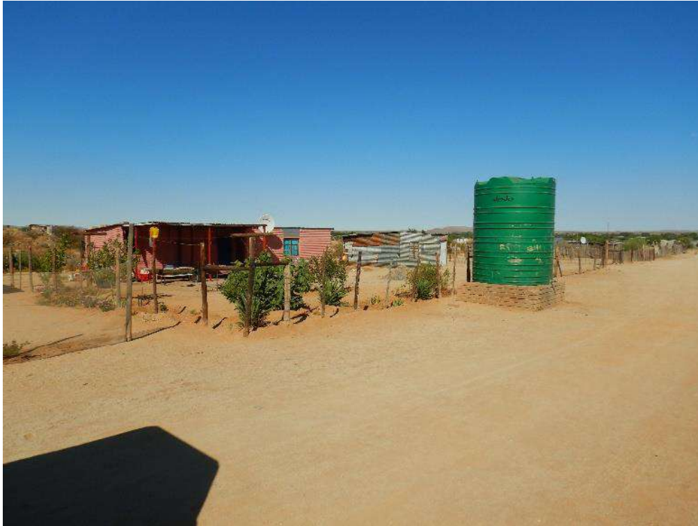
Figure 4: General view of the informal dwellings on site, looking in a south-eastern direction. The site is transformed.
