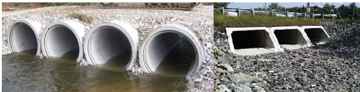
Plate 8: Installed concrete pipes and culverts (Solek, 2014)
