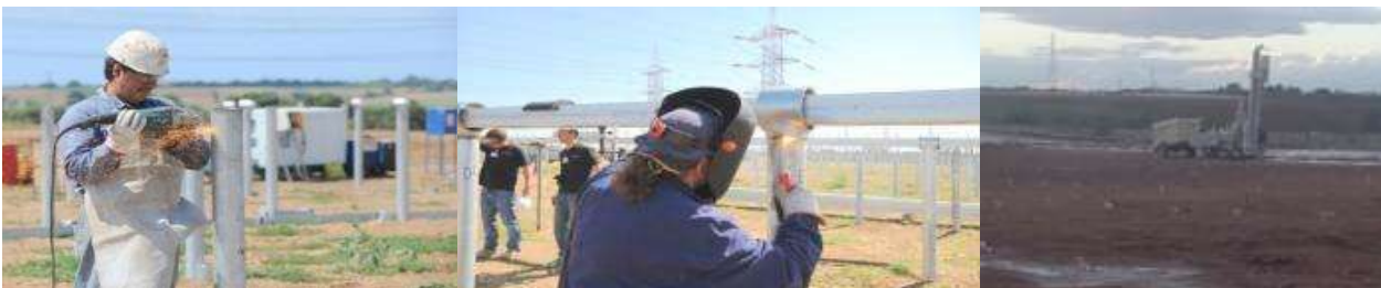
Plate 10: Showing typical erection of Solar PV modules
