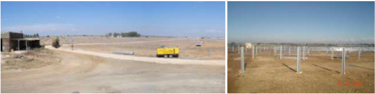
Plate 9: Typical example of site preparation activities (Solek, 2014)
