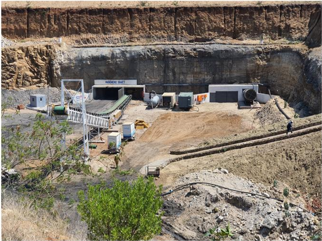
Figure 3-1: Photograph of the Mangweni Operations – Access Portal Area
