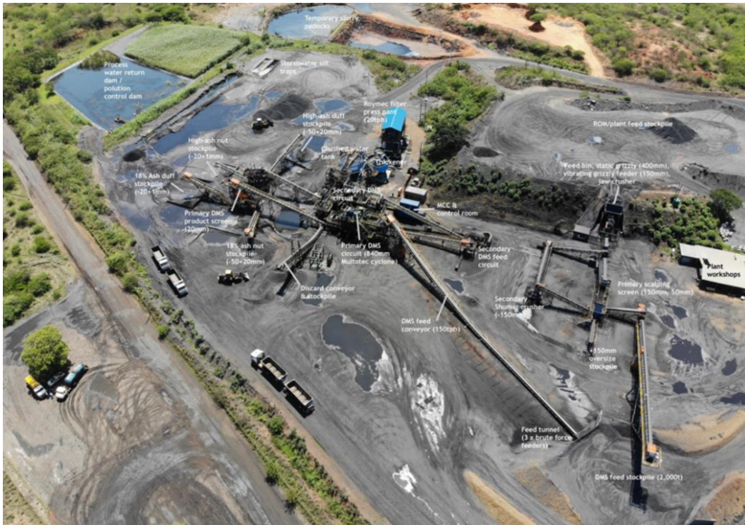
Figure 3-9: Photograph of the Beneficiation plant
