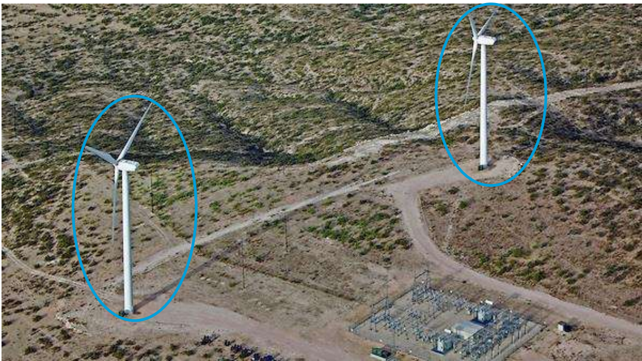
Figure 4-2: Aerial image of a wind farm in Texas 5 , which provides an indication of typical wind farm infrastructure.
