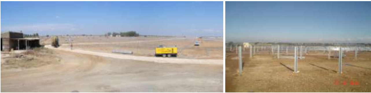
Plate 9: Typical example of site preparation activities (Solek, 2014)
