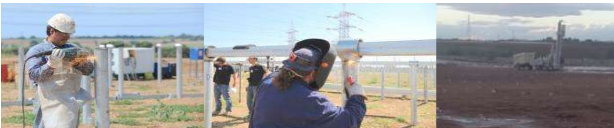
Plate 10: Showing typical erection of Solar PV modules
