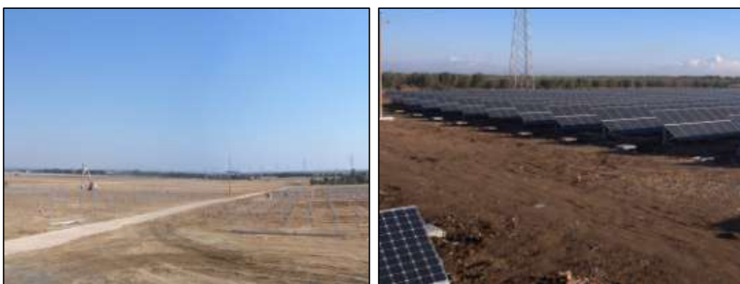
Plate 4: Showing typical example of internal access tracks (Solek, 2014)
