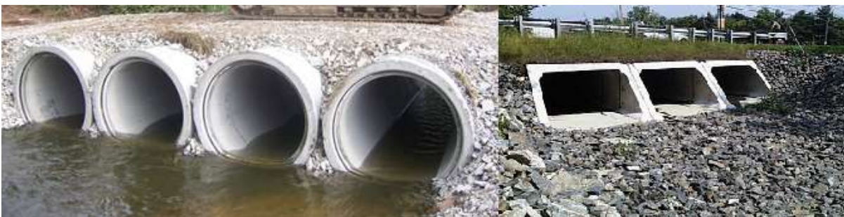
Plate 8: Installed concrete pipes and culverts (Solek, 2014)
