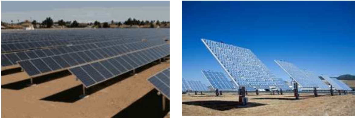
Plate 2: Showing typical examples of PV arrays (left) and CPV modules (right) (Solek, 2014)
