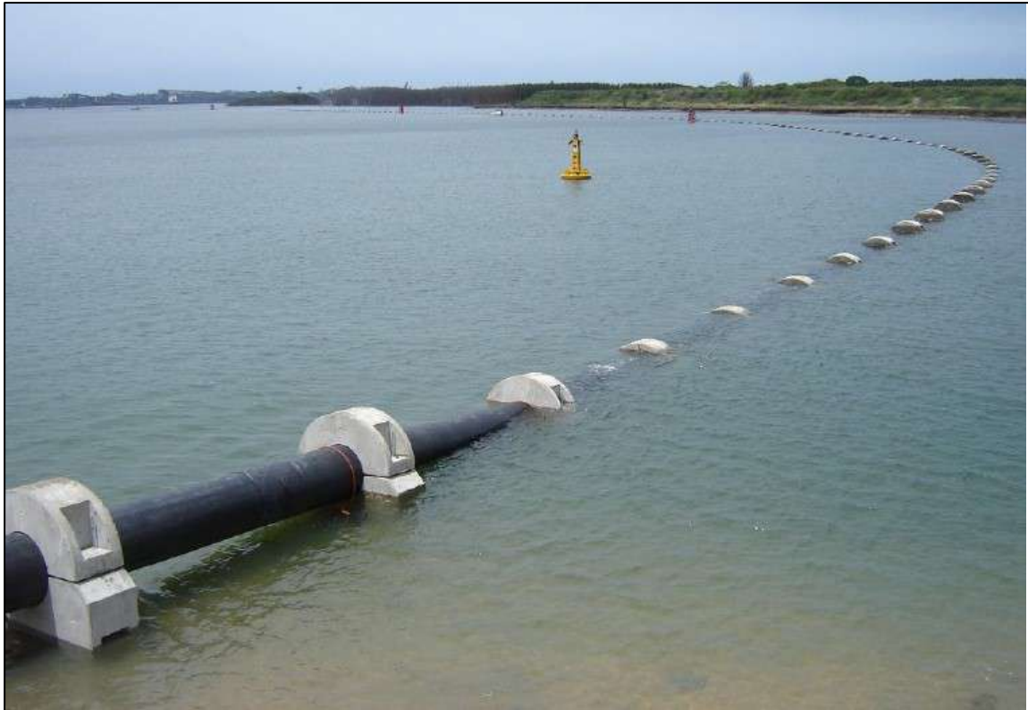
Plate 2.7: Example of HDPE pipeline with collars to provide hydrodynamic stability when placed on the seabed (WSP).
