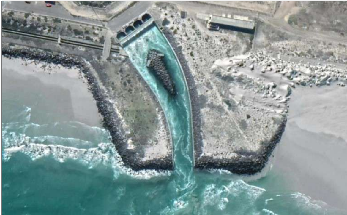
Plate 2.5: Typical outfall raceway seen at the Koeberg Nuclear Power Plant (WSP, 2020).
