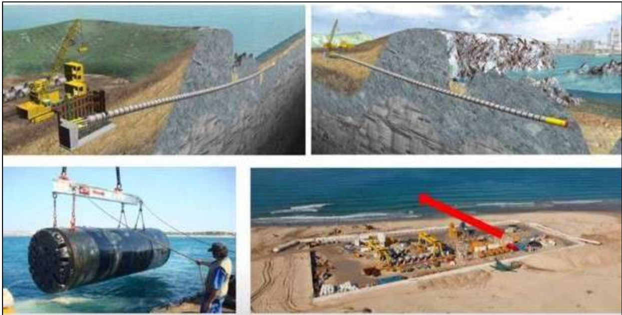
Plate 2.6: Illustration of the on-land launch shaft and jacking process during the tunnelling process (WSP, 2020).
