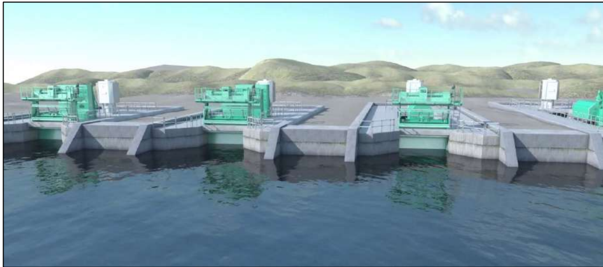
Plate 2.1: Image of cooling water intake channel configuration.
