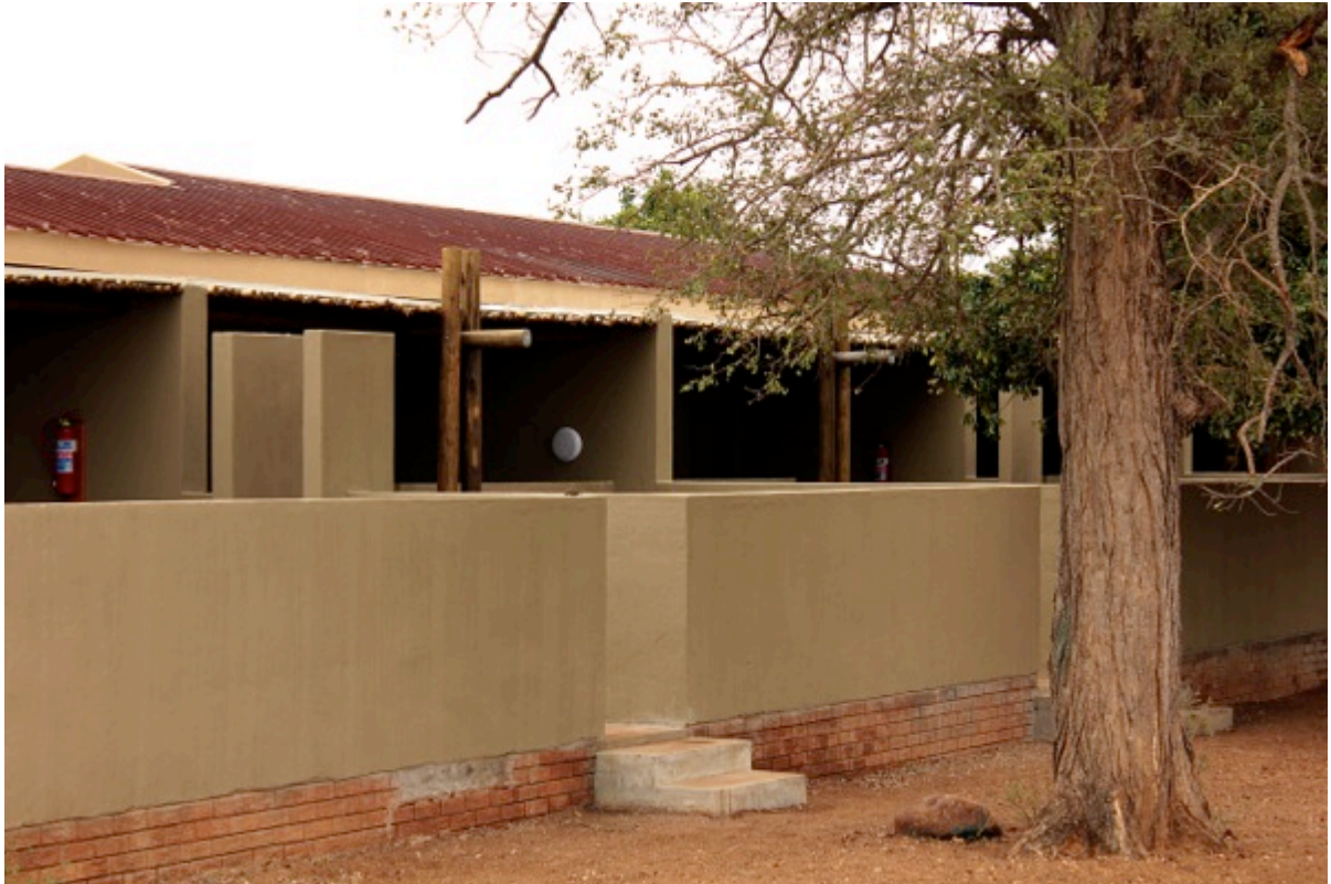
Figure 7: Other structures on the site
