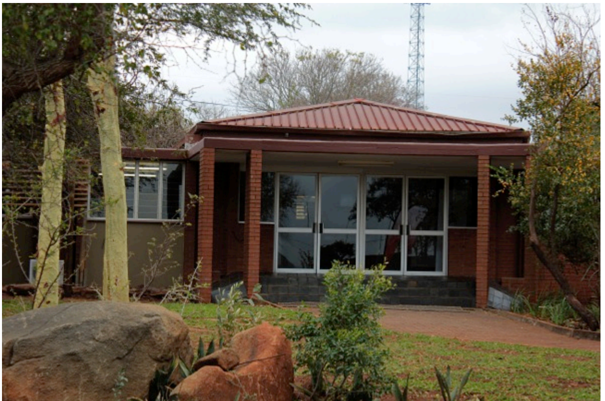
Figure 6: Recently renovated buildings on the site
