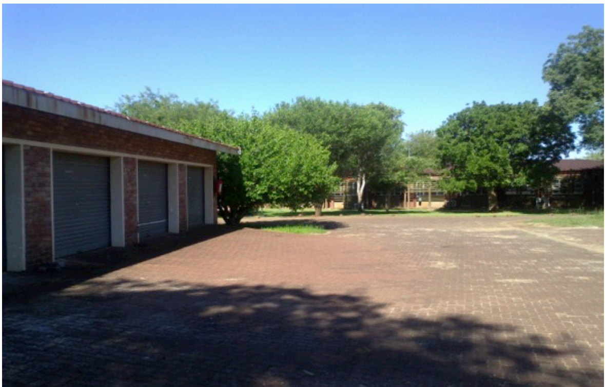
Figure 3: Disturbed vegetation around buildings and infrastructure
