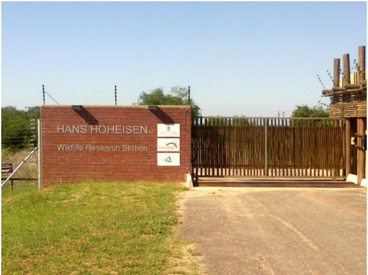
Figure 5: Access control gate to the HHWRS
