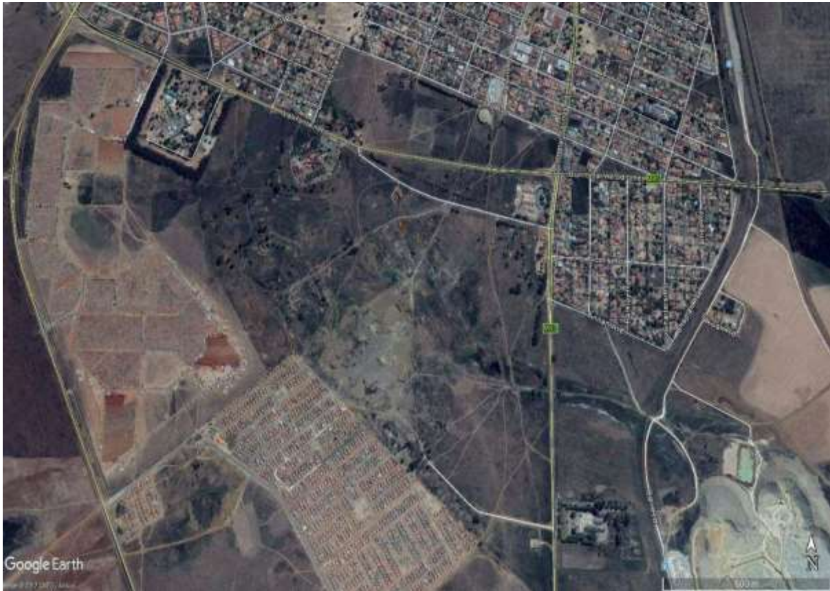
Figure 4-9: Google Earth Image of the site indicating the disturbed nature of the site
