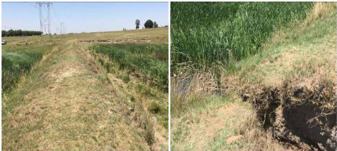
Figure 4-7: The dam wall and broken area
