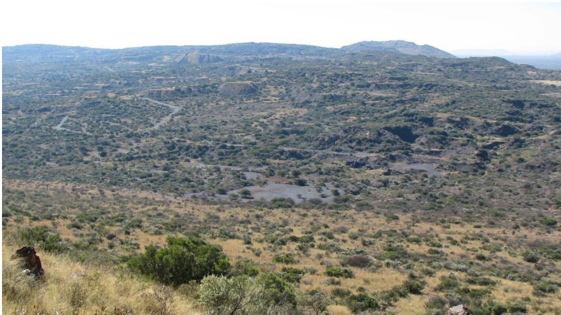
Plate 5.3.2: The effects of previous mining activity on the topography of the proposed development site.
