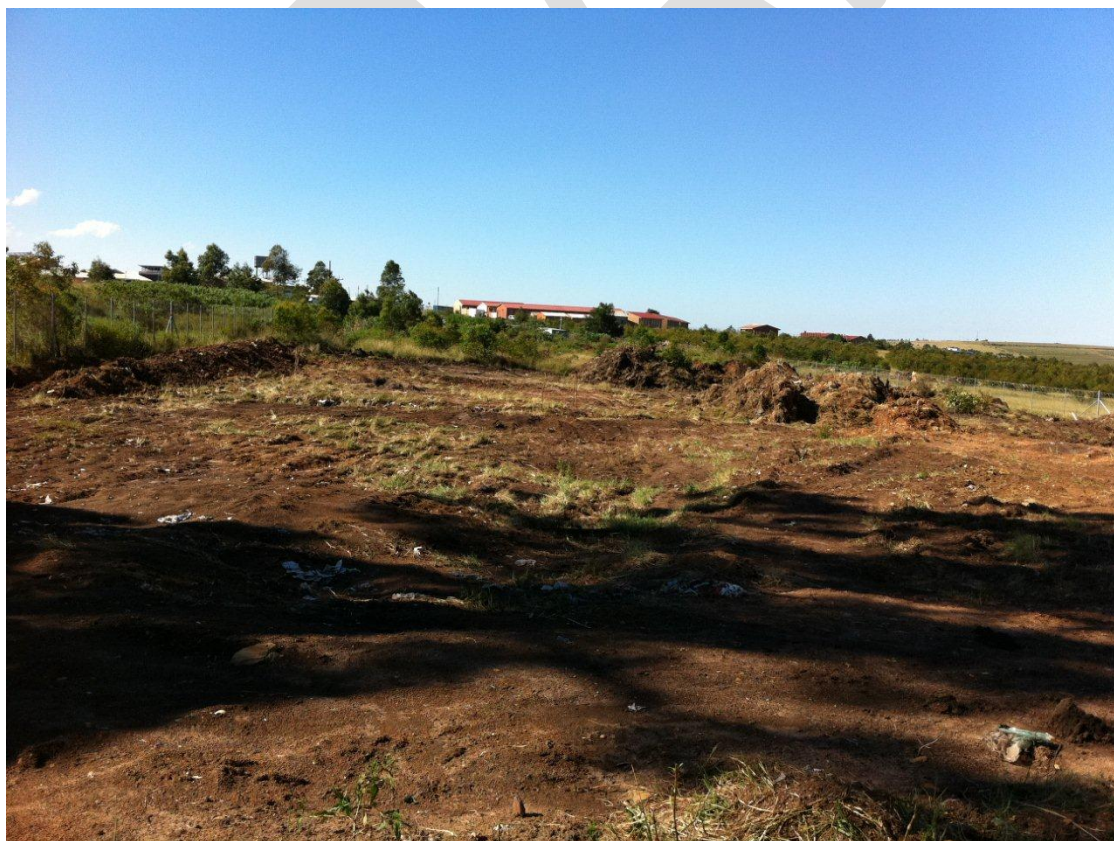
Figure 4.6 Onsite vegetation (top) and excavated site (bottom).
