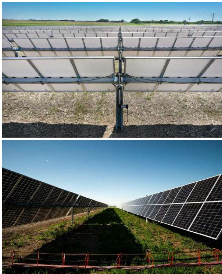
Figure 21: Monofacial (top) and bifacial (bottom) solar panels
