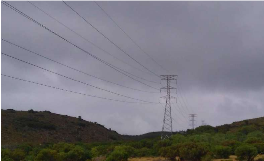
Figure 16: Example of a 132 kV transmission line
