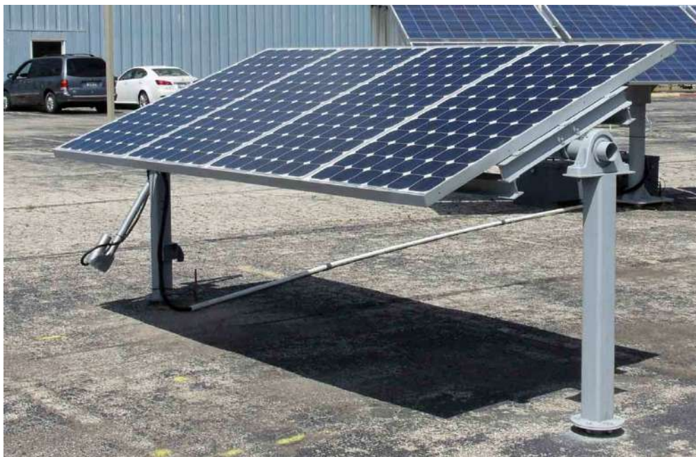
Figure 9: Example of PV Module mounted on Single Axis Tracker
