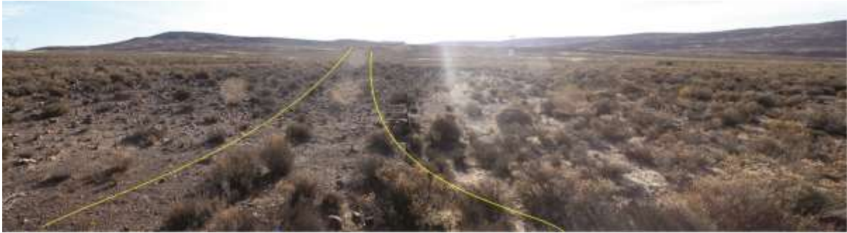
Photo 1: Photo indicating the linear dyke, looking west-north-west from the public gravel road.
