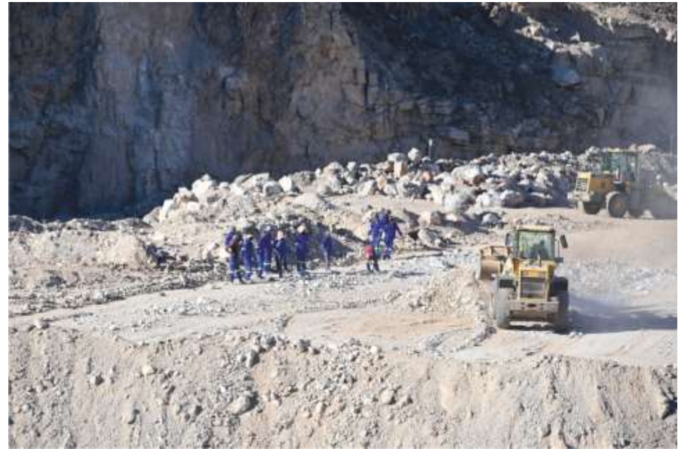
Photo 13: The sorting operation on the backfill platform. Note the safety berm before the face in the south (on the backfill platform).
