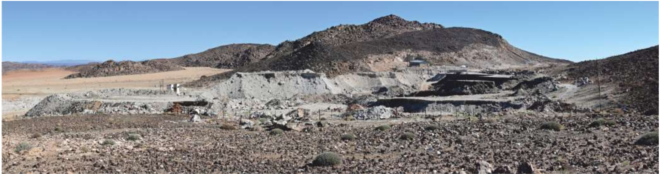
Photo 4 : Looking NE from the slope above the hostel, showing the main plant residue dump being hollowed out from the inside for re-processing and backfilling of the main section excavation.
