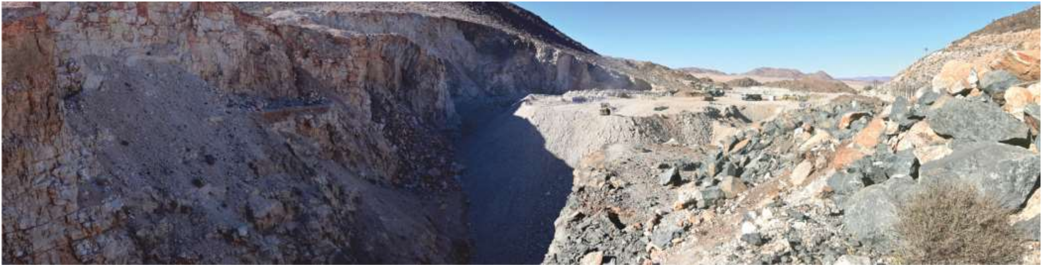
Photo 2: Looking west from the top of the Main Section excavation at the backfill which has taken place to date.
