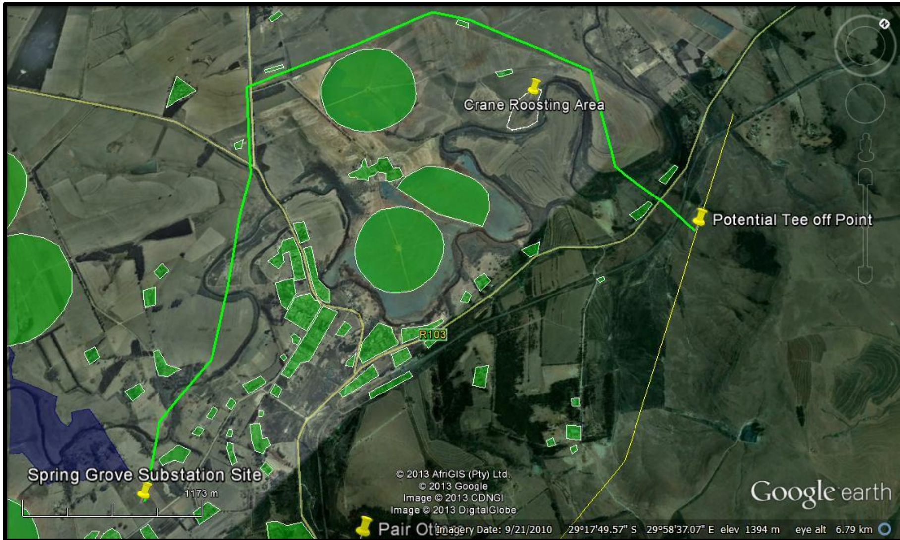
Figure 3: Aerial image of the proposed Alternative C3 88kV Powerline Servitude, KwaZulu-Natal, Fauna and Avifauna identified by the EAP during site visits has been indicated, buildings and structures have been highlight in green (Source: Google Earth 2013).
