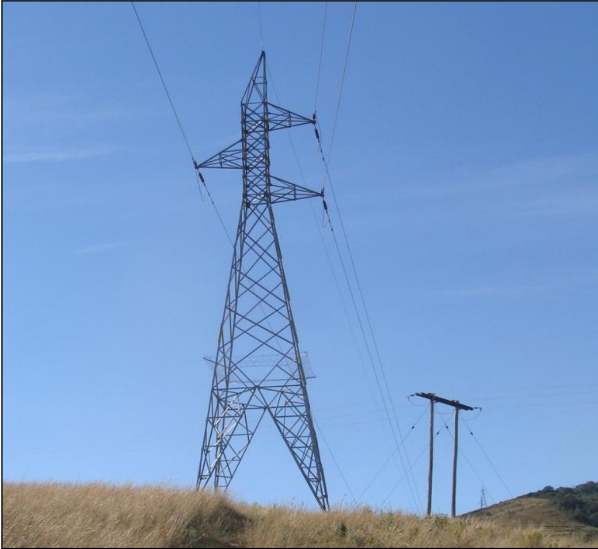
Figure 2: An example of a Single-Circuit 88KV self-supporting tower type that is the second design Alternative for the Spring Grove Tee powerline.
