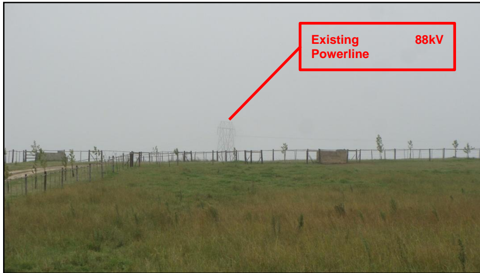
Figure 1: Existing 88kV Powerline that the proposed Spring Grove Tee will connect to.
