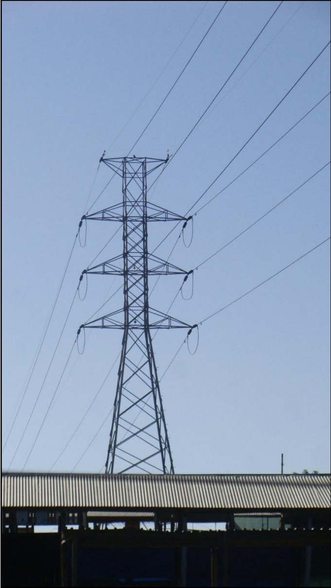
Figure 1: An example of the Double-Circuit 88KV self-supporting tower type that is the preferred design Alternative for the Spring Grove Tee powerline.
