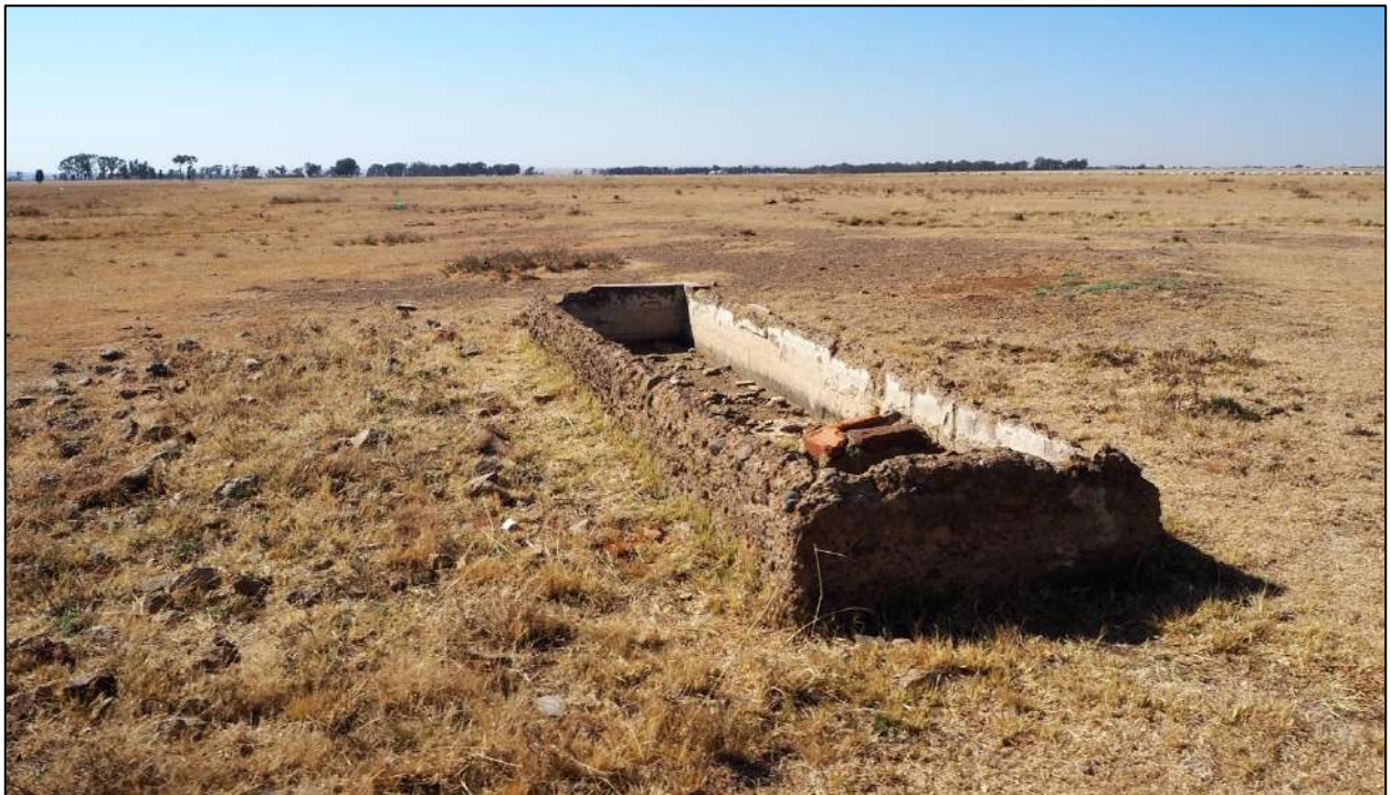
Figure 20. Troughs close up
