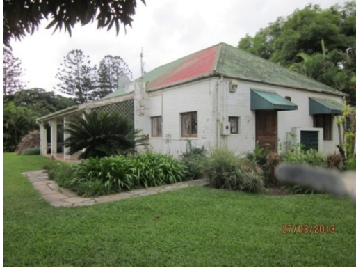
Fig 24: South west corner
