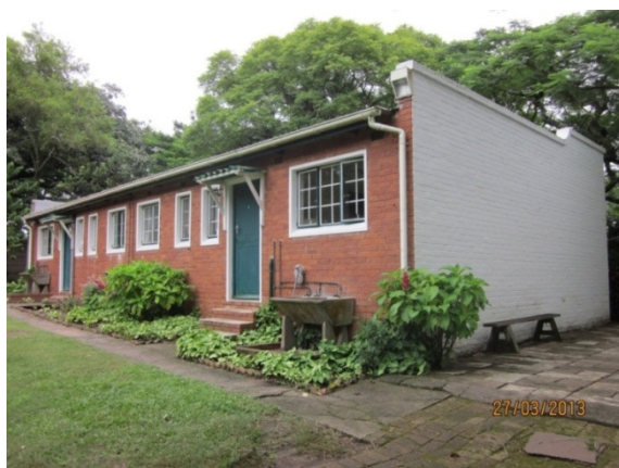
Fig 11: Staff quarters from Labour compound
