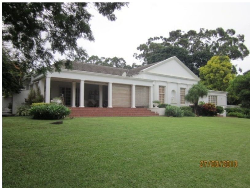
Fig 5: North western façade
