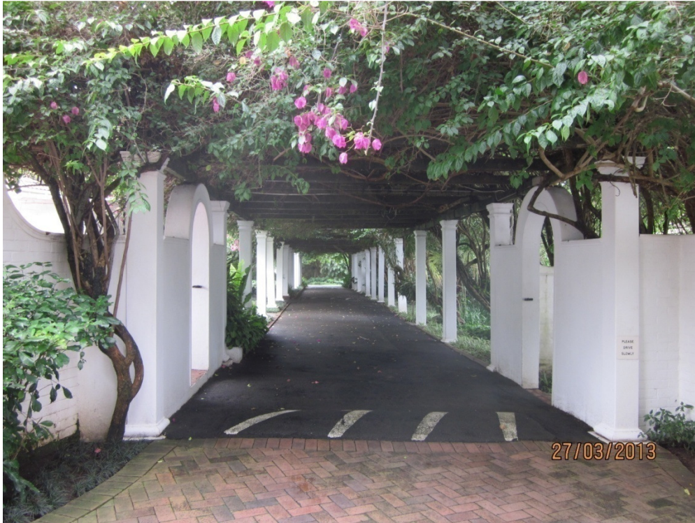
Fig 1: Pergola entrance to Herrwood House
