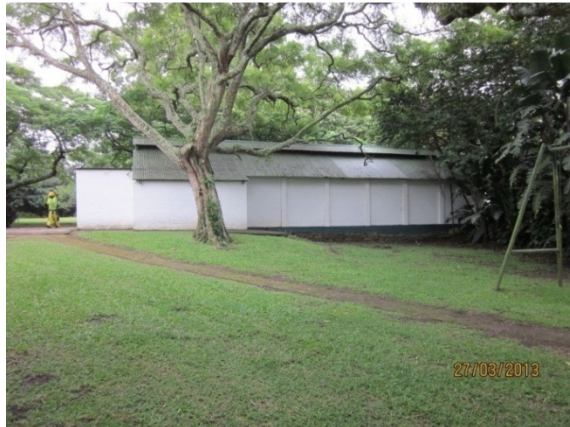
Fig 10: Stables from south east showing stone foundations
