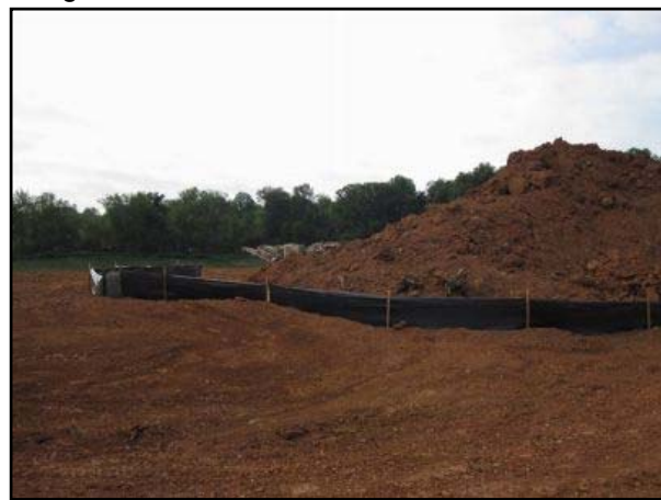
Figure 21: Silt fences protecting controlling erosion around a stockpile (source: www.tnepsc.org)
