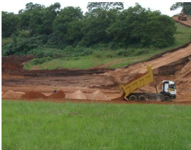
Figure 16: An example of soil that has been stockpiled in a designated stockpile area on flat ground near to minimize runoff and impact on the surrounding environment.
