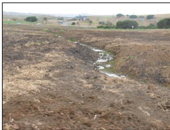
Figure 26: Wetland system draining water towards the north-east corner of the site.
