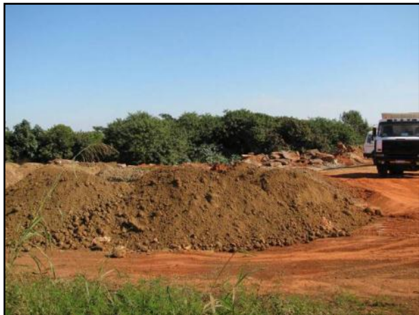
Figure 18: An example of a legal spoil site used during the construction of a road.
