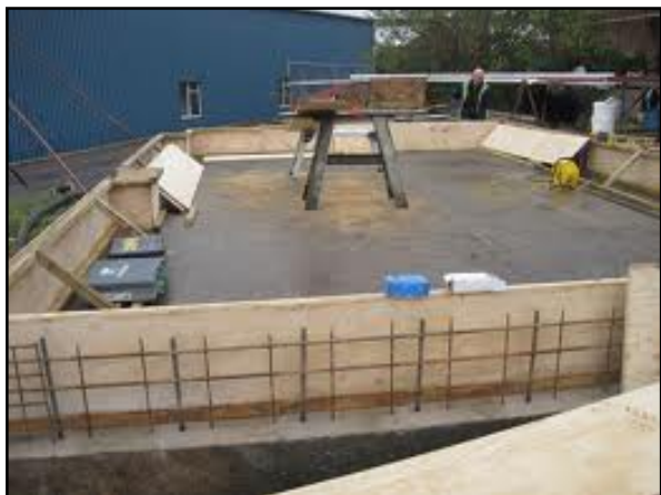
Figure 4: An example of a bunded area that should be used to contain the hazardous store area within the construction camp (Source: www.oasis-environemts.co.uk ).
