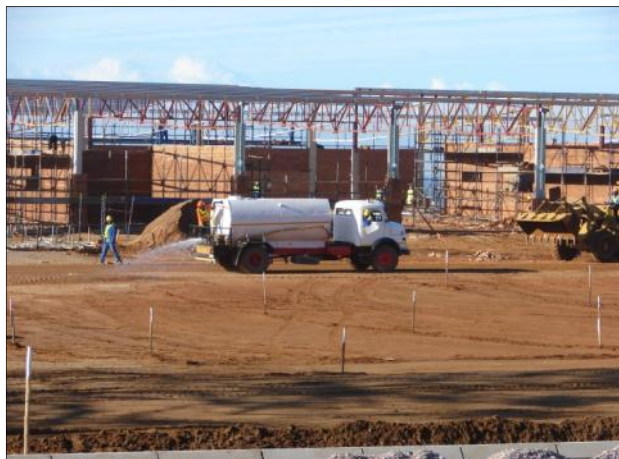
Figure 30: An example of dust suppression at a construction site to control dust generation.
