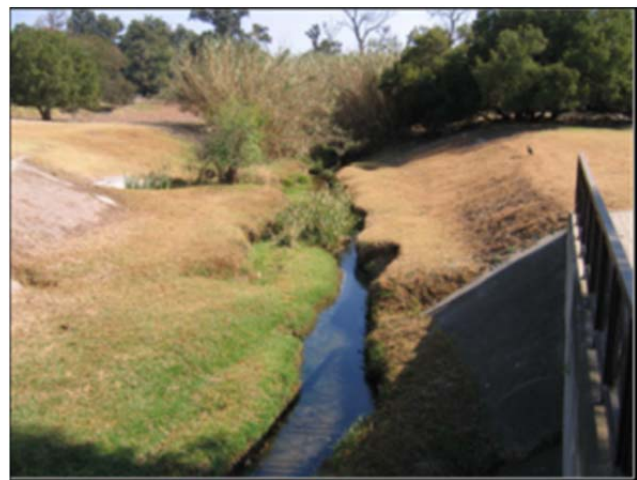
Figure 8: Example of a “formalized” stormwater drain taking the environment into consideration (Source: Wetland Impact Assessment, April 2013, WetCS)
