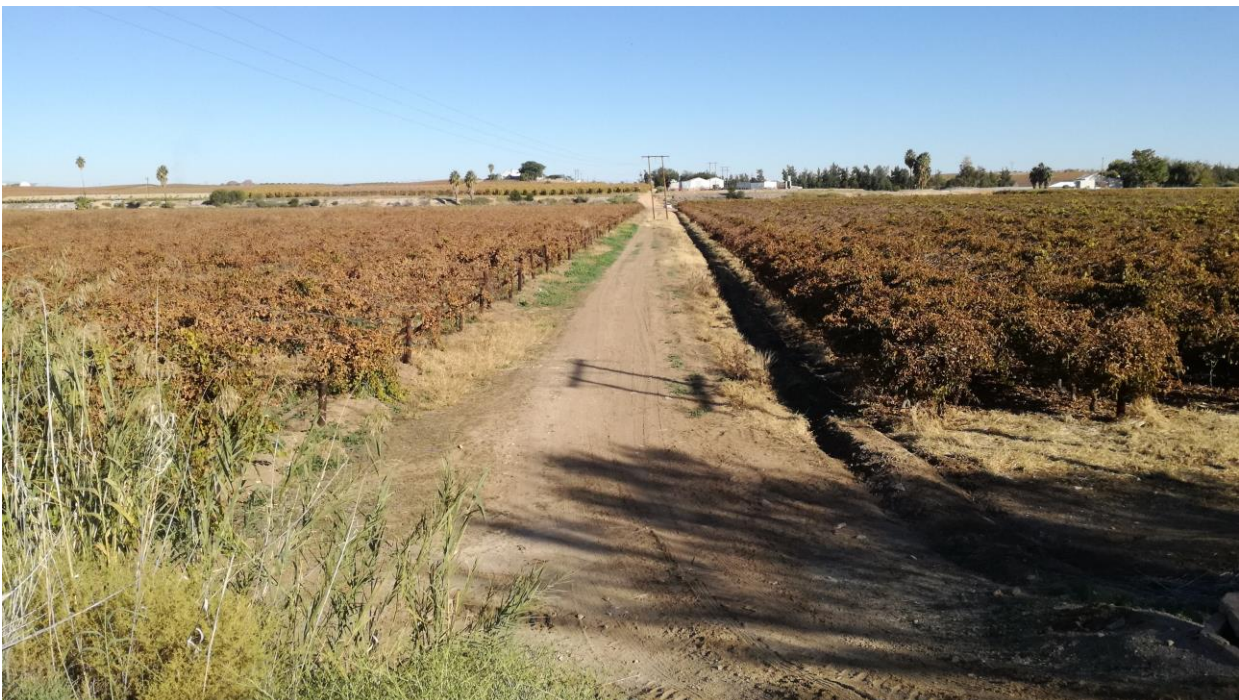
Figure 5: General view of part of the pipeline route (along the existing track). This is located within a registered servitude. Also note the existing vineyards, typical of the dominant land-use of the area.
