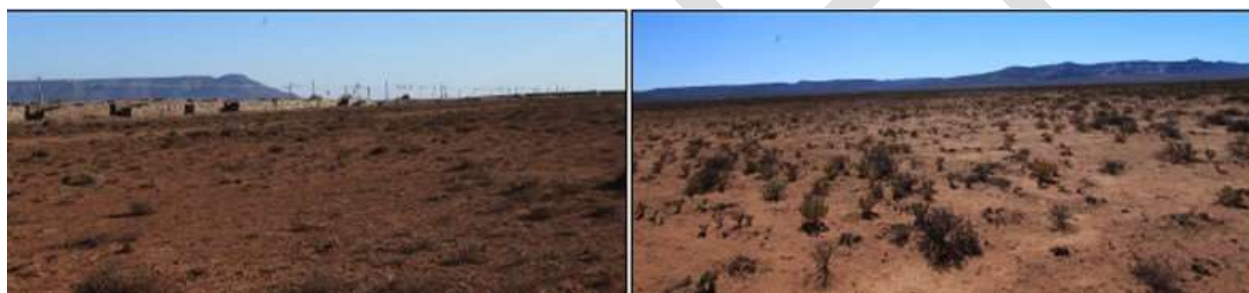
Figure 17: General view of the proposed open cast and infrastructure areas, indicating the Transnet railway line, limited vegetative cover, bare ground, relatively flat topography of the area, with mountains in the greater region (Scientific Terrestrial Services, July 2018e)
