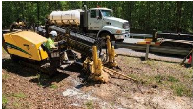
FIGURE 5: A TYPICAL ILLUSTRATION OF DIRECTIONAL DRILLING.
