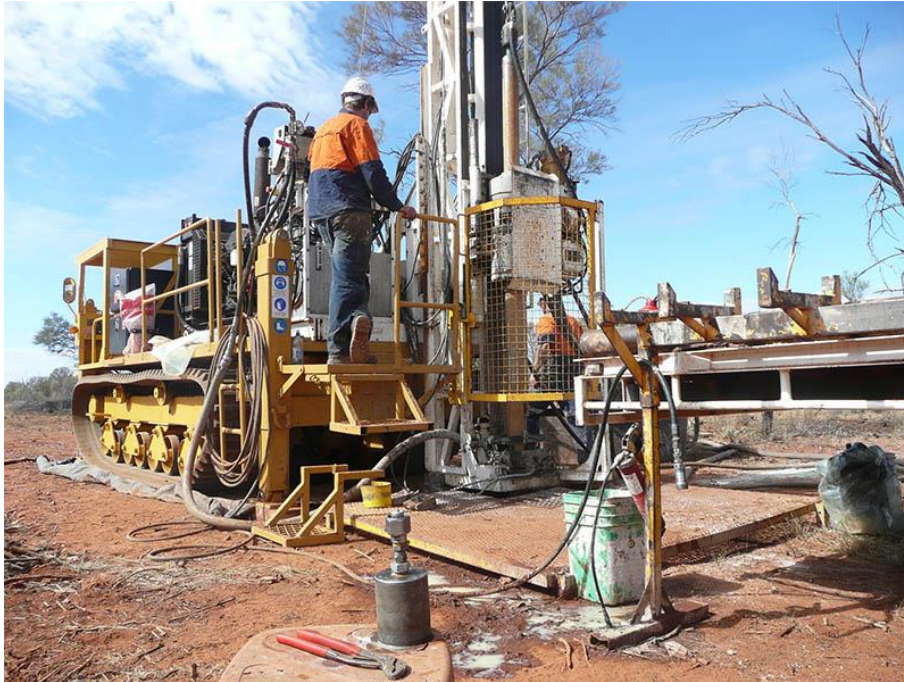
FIGURE 6: A REVERSE CIRCULATION DRILL RIG.
