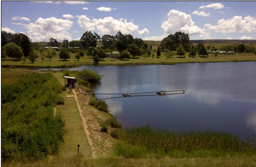
Figure 2-1 : Dullstroom Dorp se Dam : looking from left abutment to right bank caravan park
