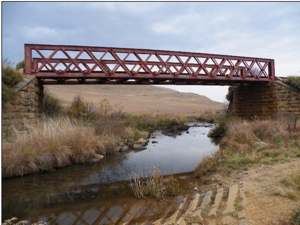
Figure 8-2 : Rail bridge from upstream
