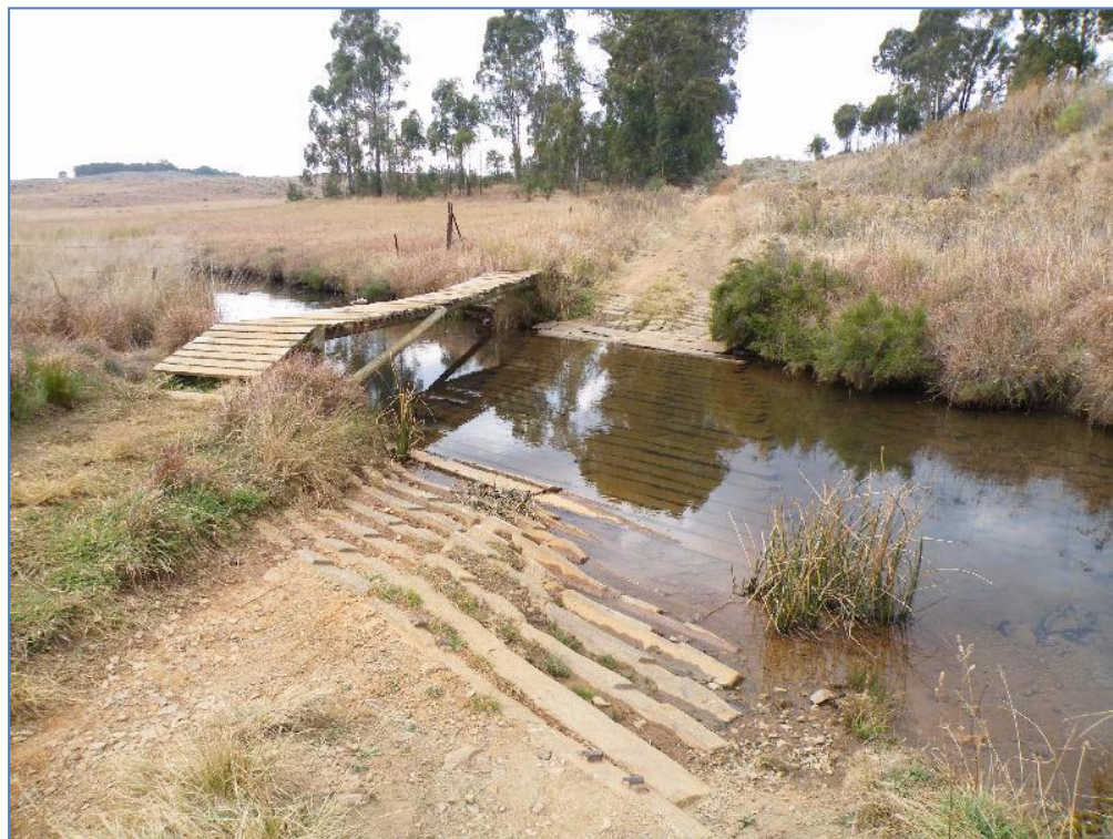
Figure 8-4 : Service road drift and upstream footbridge
