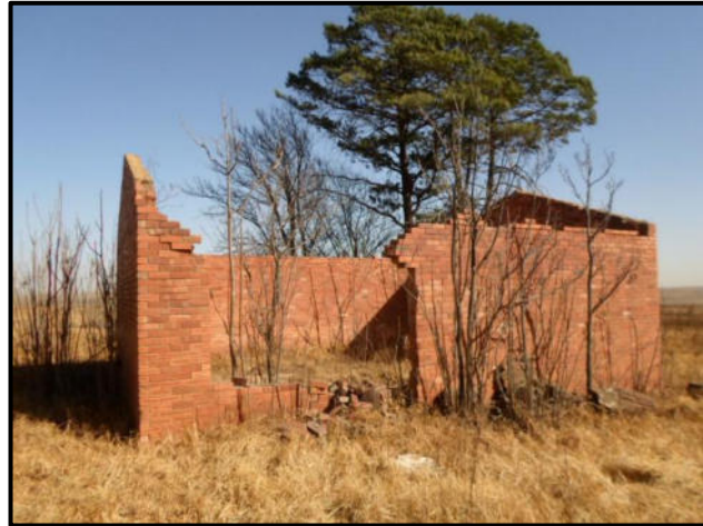
Figure 7-64: Red brick structure viewed from the west
