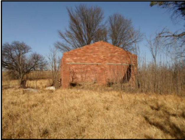
Figure 7-63: Red brick structure viewed from the north
