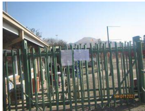
Plant Entrance (Project 4 and 5)
