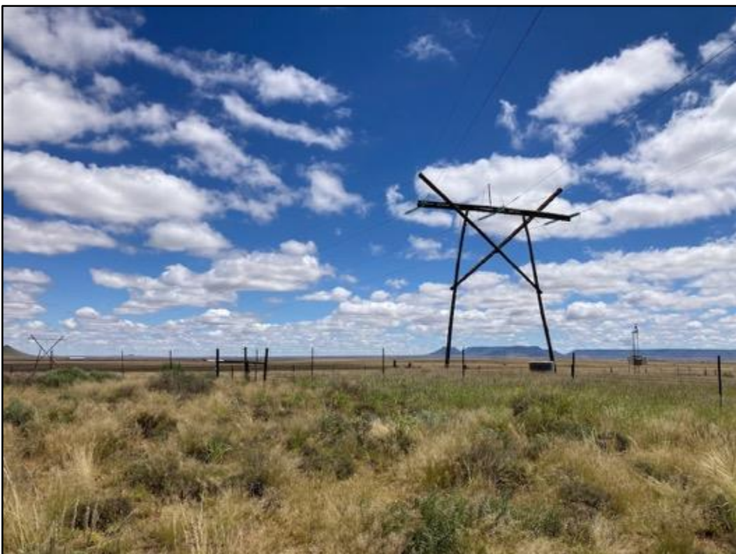
Figure 8: View of corridor at northern end.
