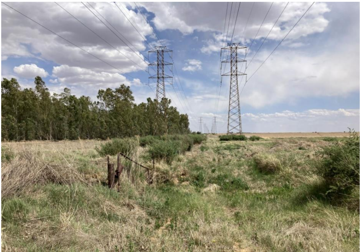
Figure 3: High voltage lines in the assessment area
